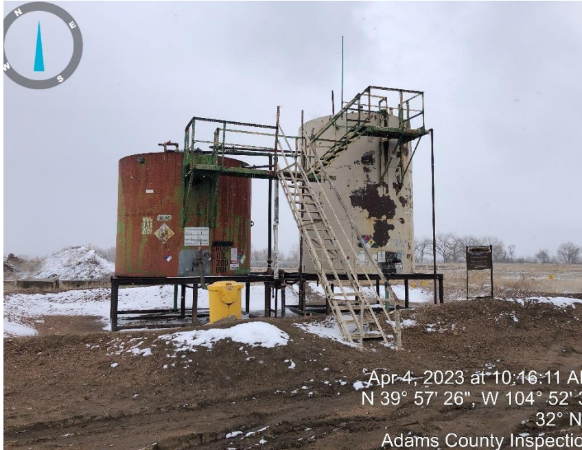
Photo# 1 Crude Tank and P/W Tank.
