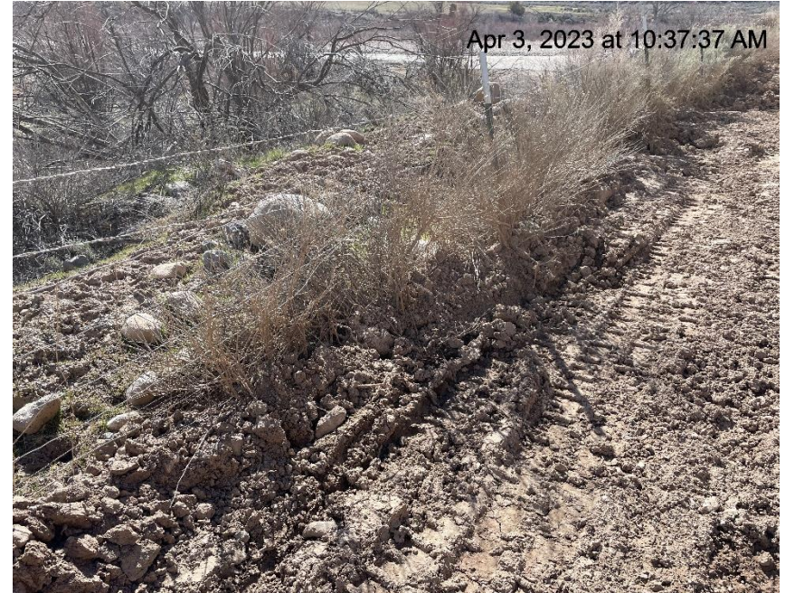
Photo # 4022 Transport of sediment/insufficient BMP's (approximately 1.7 miles down lease road)
