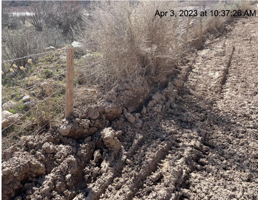
Photo # 4021 Transport of sediment/insufficient BMP's (approximately 1.7 miles down lease road)
