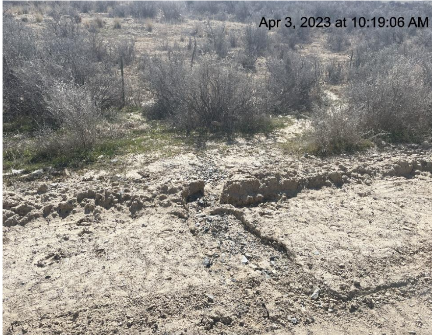
Photo # 3997 Rill erosion & transport of sediment off lease road (approximately 1.5 – 1.6 miles down lease road)
