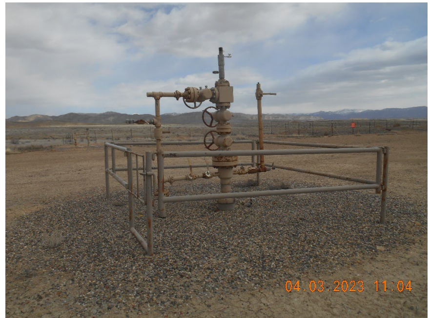
Wellhead Temporarily Abandoned
