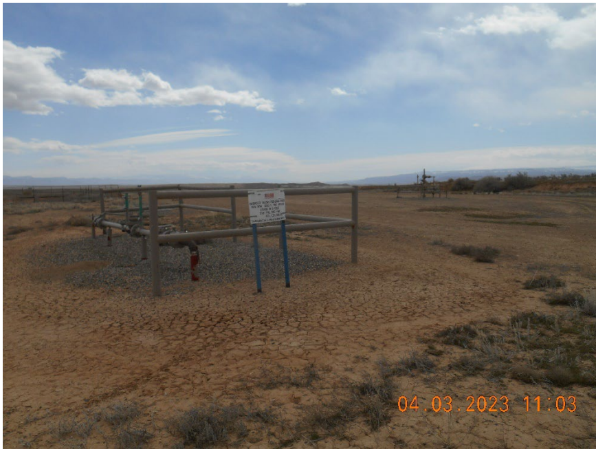
Location overview looking SE.
