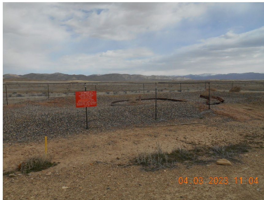
Tank battery. Tanks removed.
