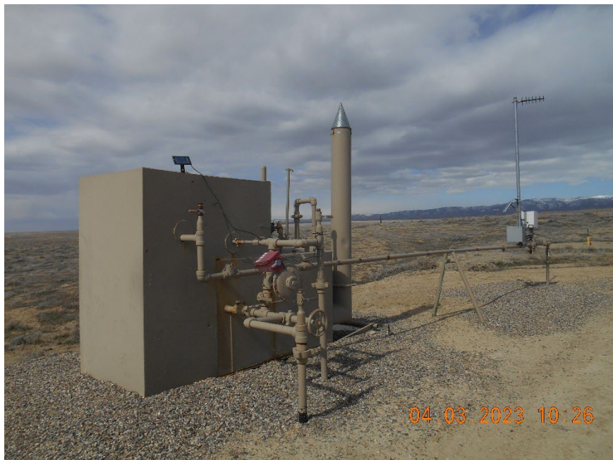
Separator with meter
