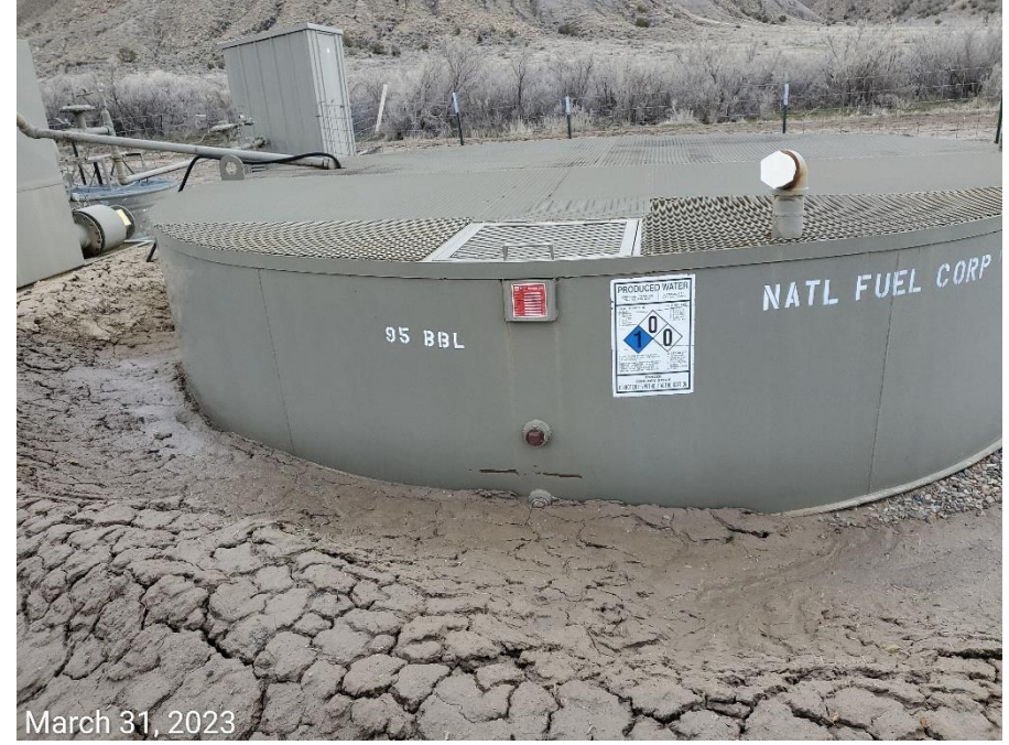
Photo 3: Tanks on Location- Labels missing required information per Rule 605.h.
