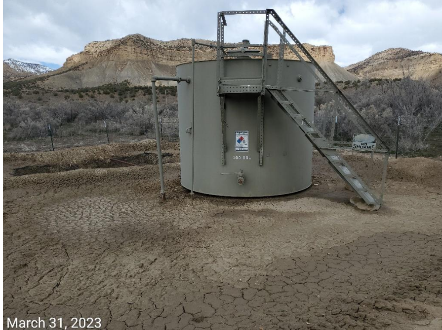
Photo 3: Tanks on Location- Labels missing required information per Rule 605.h.
