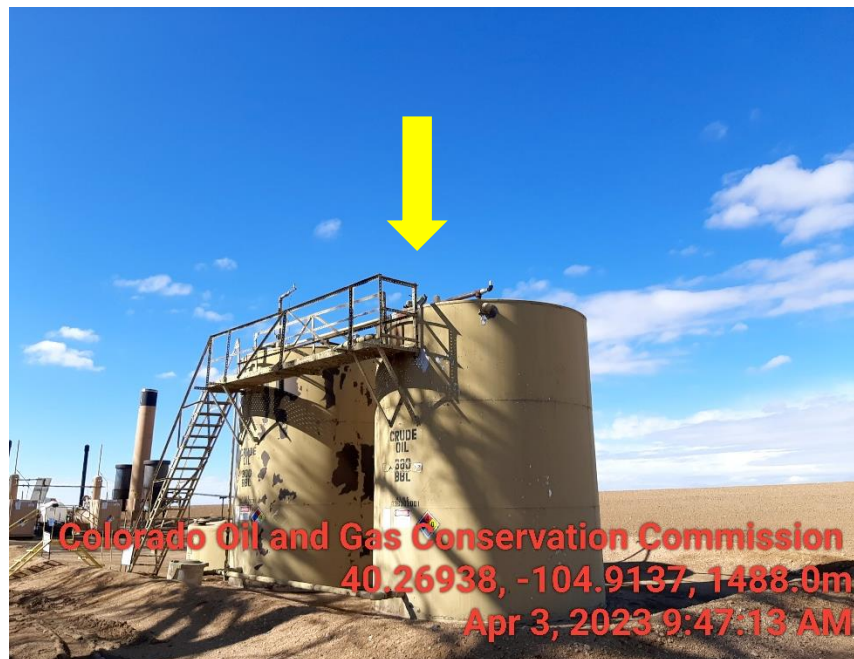
Photo 1 Gauge hatch open
