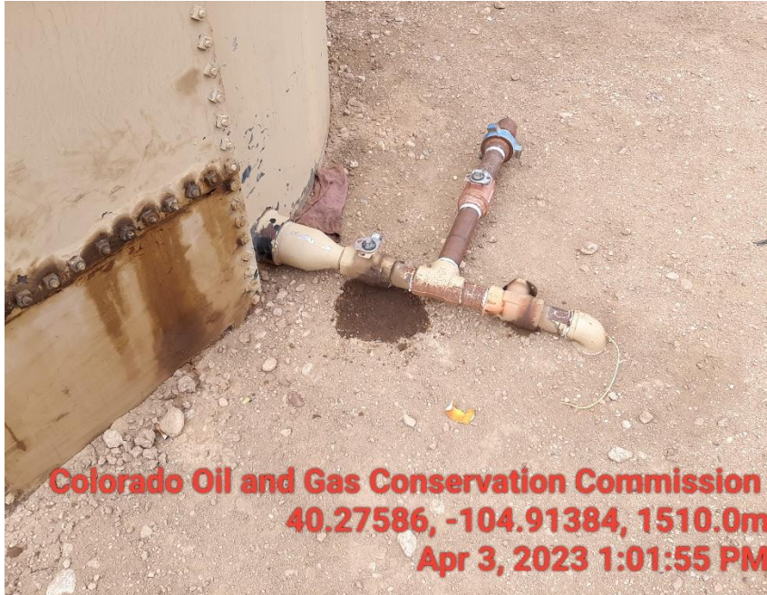
Photo 1 Stained soil 2" line on crude oil tank.
