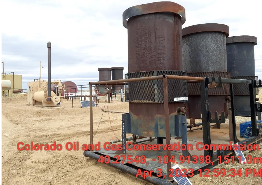
Photo 11 portable EDC unit hooked to line from Crude oil tanks.
