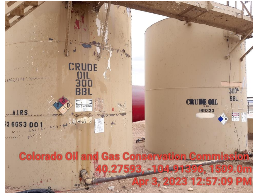
Photo 6 NFPA placards faded on crude oil tanks
