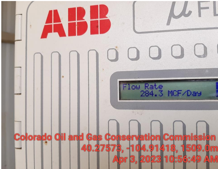
Photo 9 Meter station 235486 showing production
