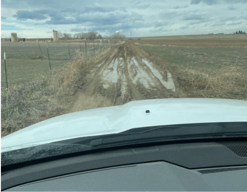
Photo 13 Roads deep ruts and holding water.
