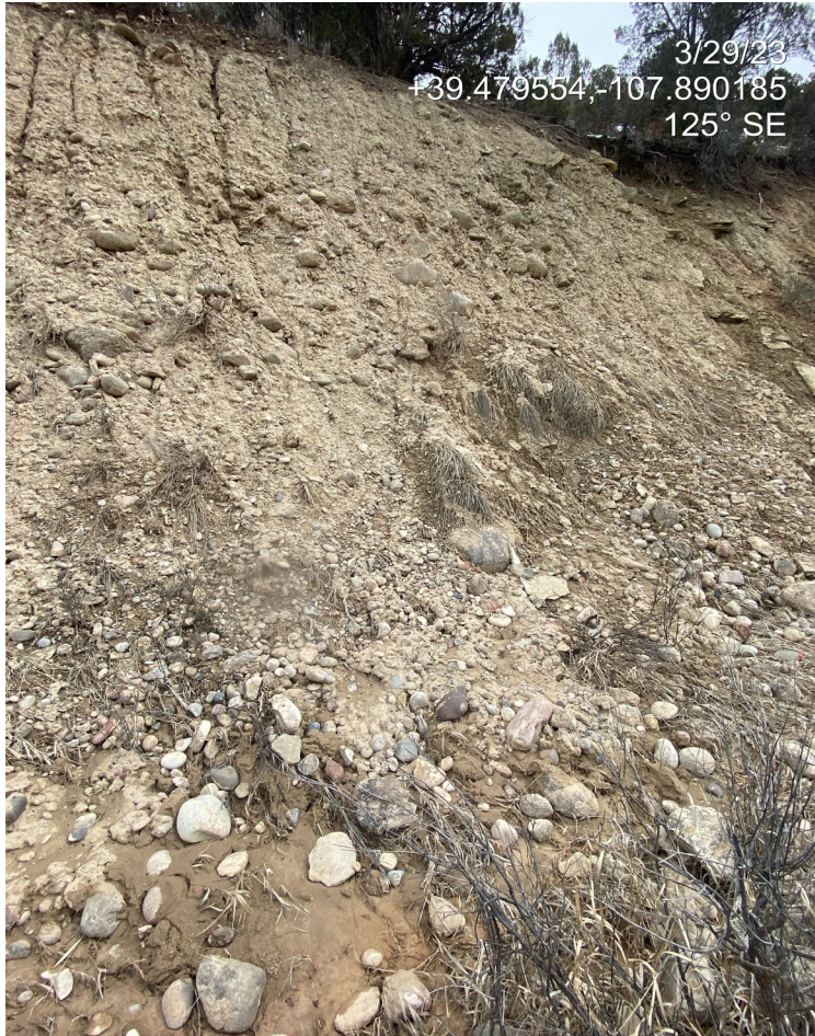
Photo 6. Photos show sediment accumulating at the base of the eastern cut slope. Erosion is resulting in degradation to the slope, smothering vegetation below and contributing sediment loads to stormwater.
