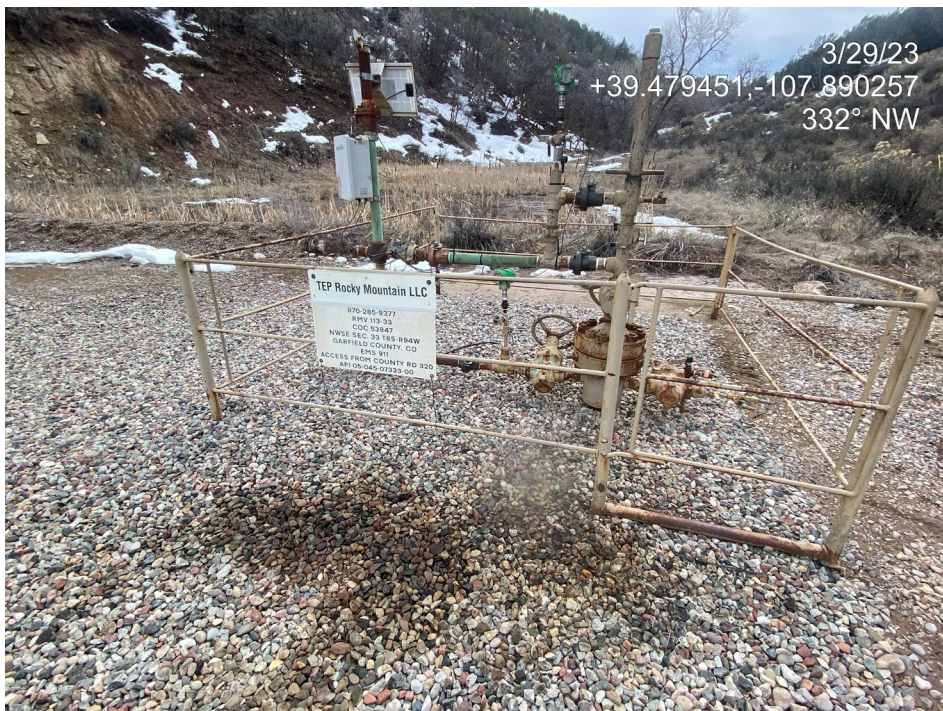
Photo 2. Photos show production areas. Note stained gravel at the wellhead (left).
