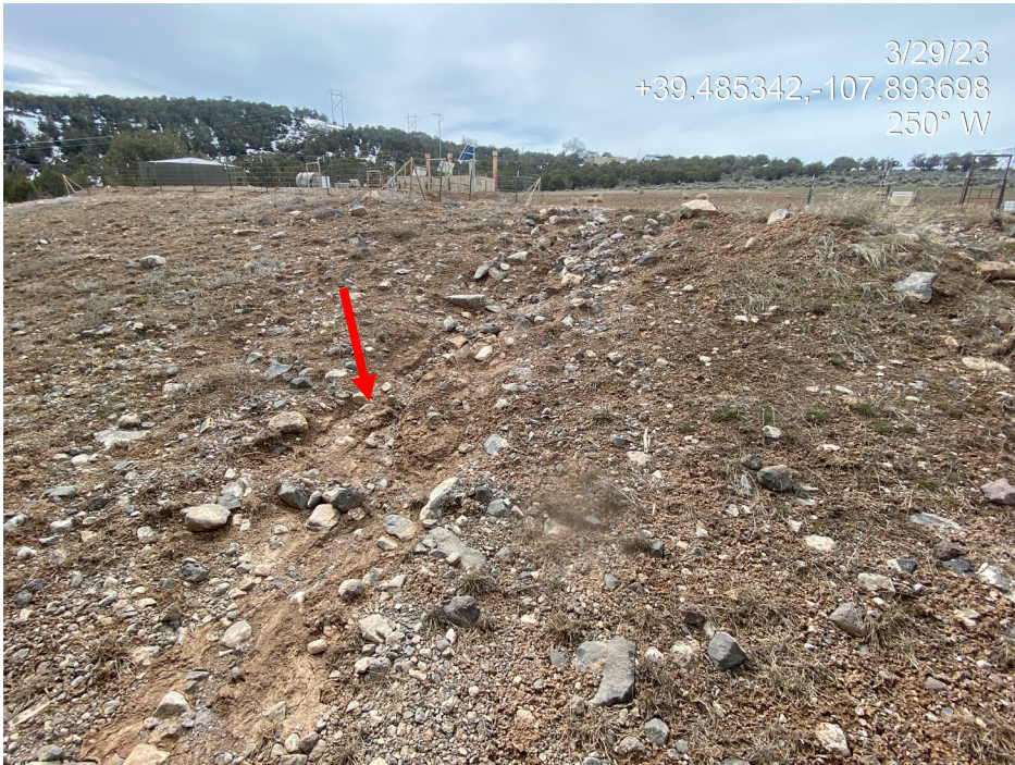
Photo 5. Photos show an example of rill erosion on the fill slope to the east of the location (left) continuing offsite into reference areas in the form of rill erosion and sediment deposition (right).
