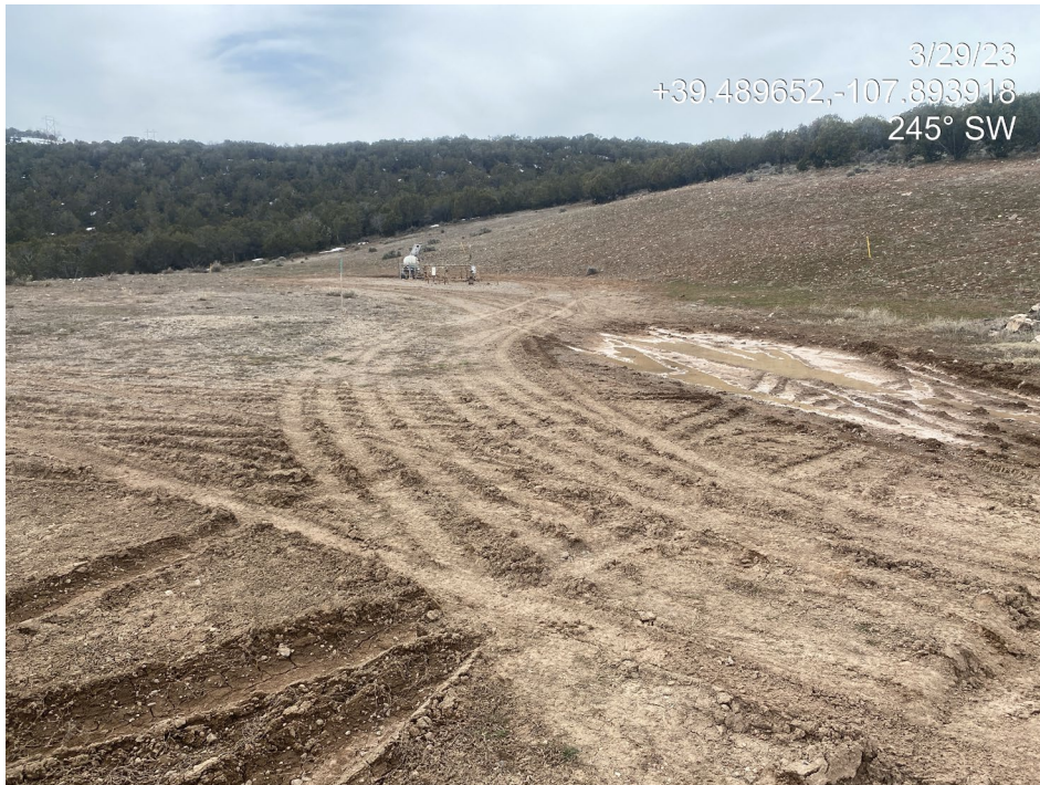
Photo 1. Photos taken from the entrance shows an overview of the upper/northern portion of the location (left) and production areas (right). Note lack of stabilization/compaction (ruts).
