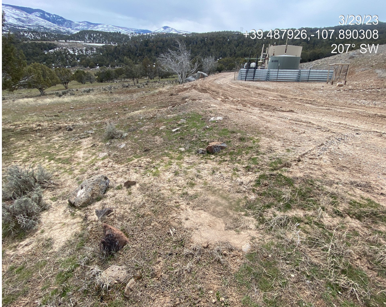
Photo 3. Photo shows the southern/lower production area. Note the unstabilized access road and erosion and sediment deposition to the south/left of the road.
