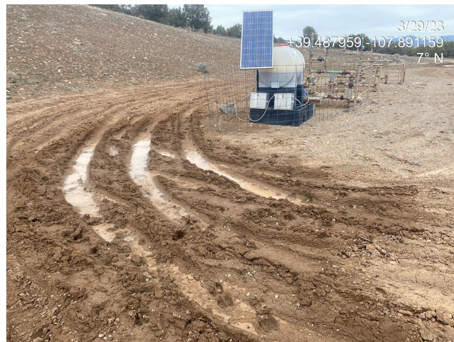
Photo 1. Photos taken from the entrance shows an overview of the upper/northern portion of the location (left) and production areas (right). Note lack of stabilization/compaction (ruts).
