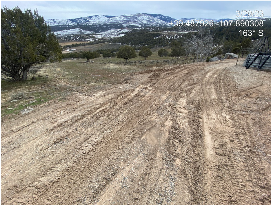
Photo 5. Photos show lack of stabilization of the access road.
