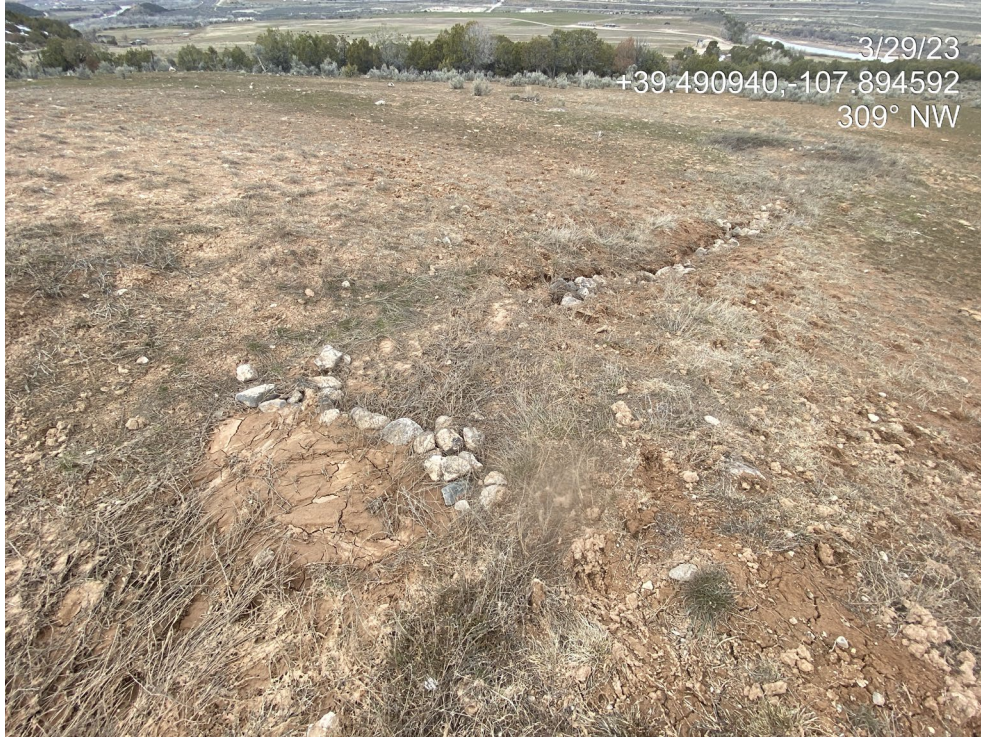
Photo 8. Photo shows an overview of the northern interim area including a stormwater ditch/slope drain. Northern interim areas are partially vegetated, however, erosion degradation is present.
