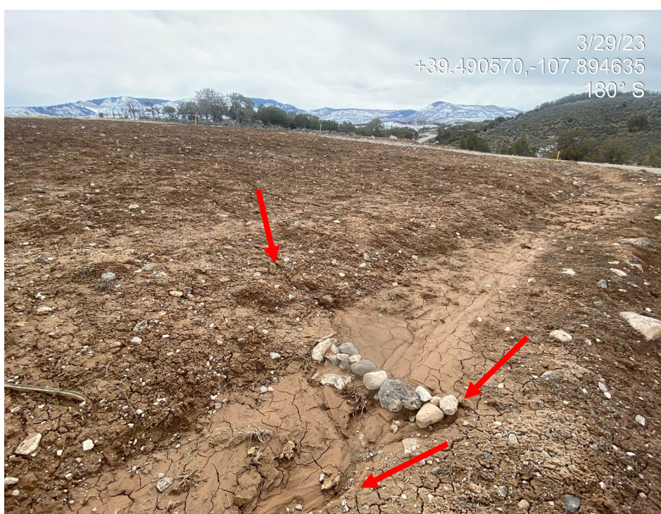
Photo 5. Photo shows the stormwater ditch at the south of the location is full of sediment lost from the southern interim area. Note rills in interim area and degradation to the stormwater ditch and rock check dam.
