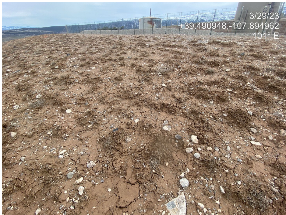
Photo 10. Photo shows pedestaling around vegetation in the northern interim area indicating erosion.
