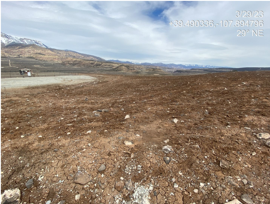
Photo 4. Photos show soils in the southern interim area are bare and unstabilized (left) resulting in rill erosion (right).
