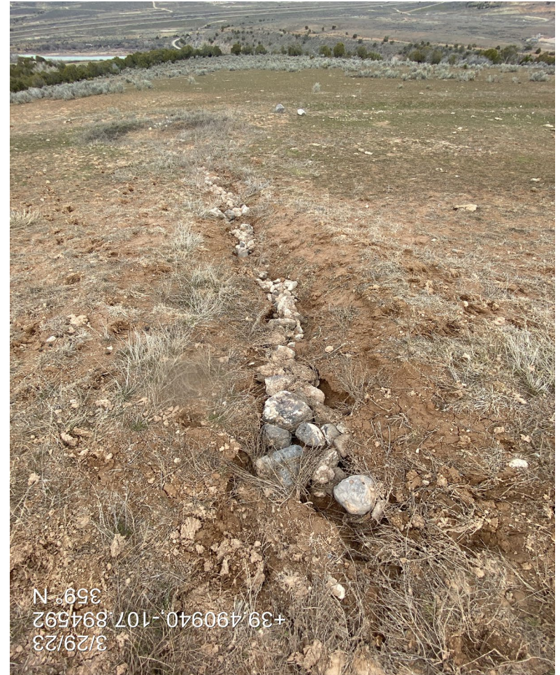
Photo 9. Photo shows degradation in the stormwater ditch/slope drain at the north of the location.
