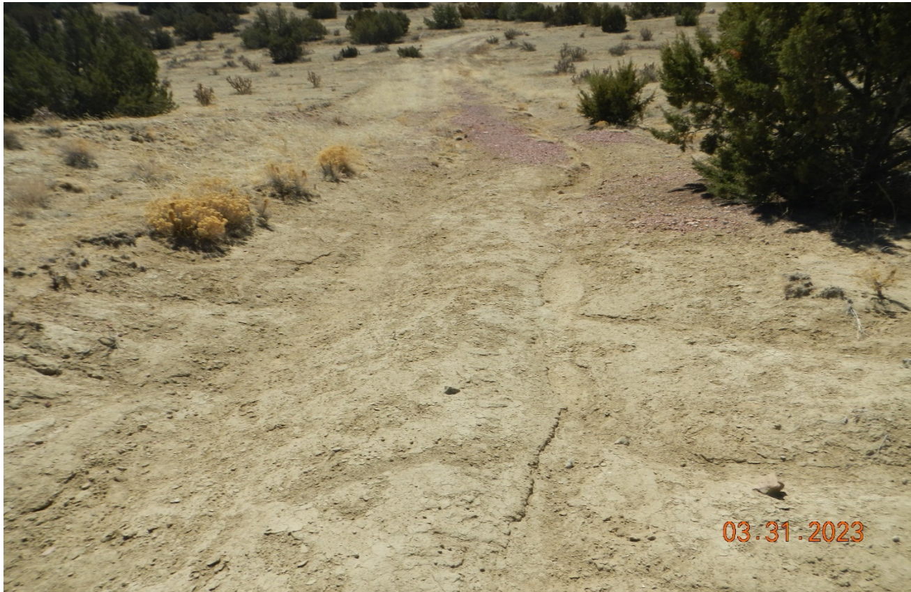
Photo 2. There is erosion along this area of the road which needs to be repaired and stabilized. Previous corrective action was not performed.
