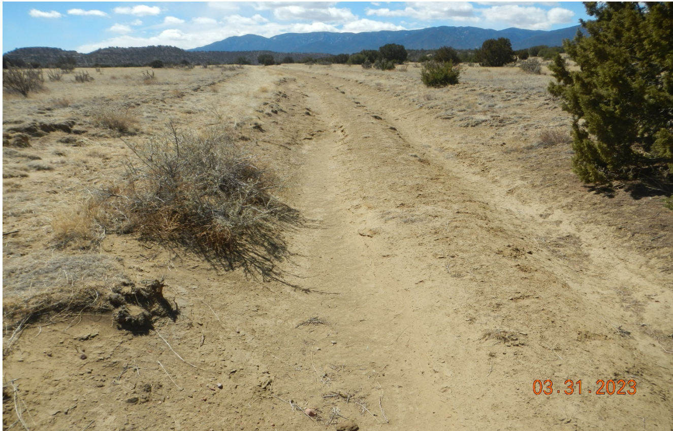
Photo 1. Facing south along the preexisting portion of the road. There is erosion and deep vehicle ruts along the road that have not been repaired and stabilized. Previous corrective action was not performed.
