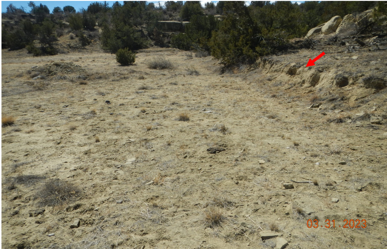
Photo 6. There is a cut into the embankment which has not been recontoured and reclaimed..
