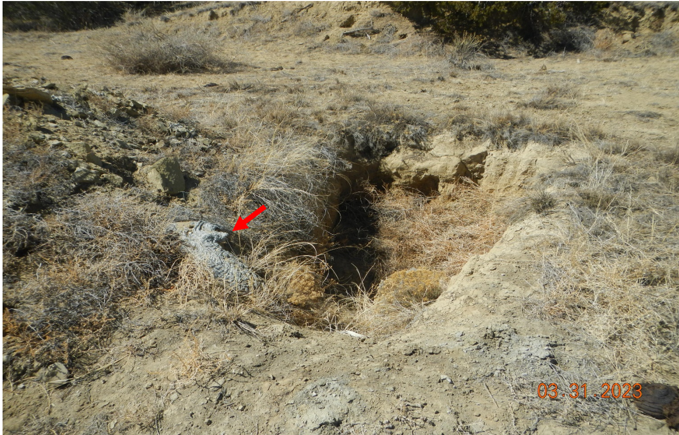
Photo 5. There is an open hole that is about 4.5 ft. deep. There is cement debris next to the hole which appears to be from plugging of the well. Previous corrective action has not been completed.
