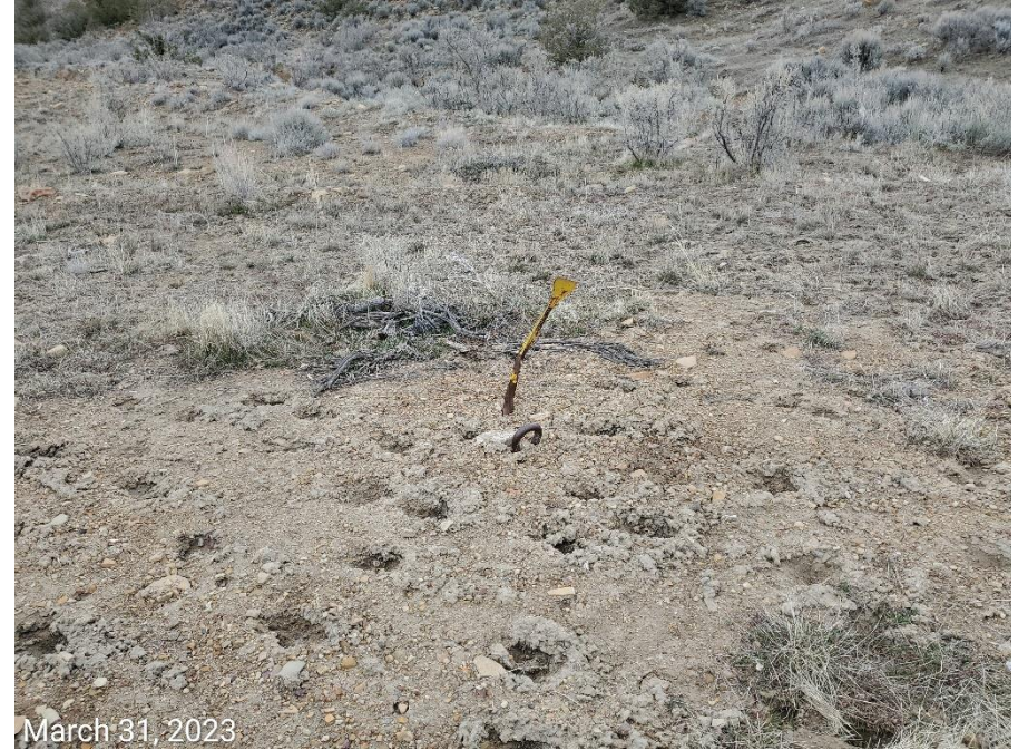
Photo 4: Photos examples showing anchor markers are either missing, or inadequate per Rule 1003.a
