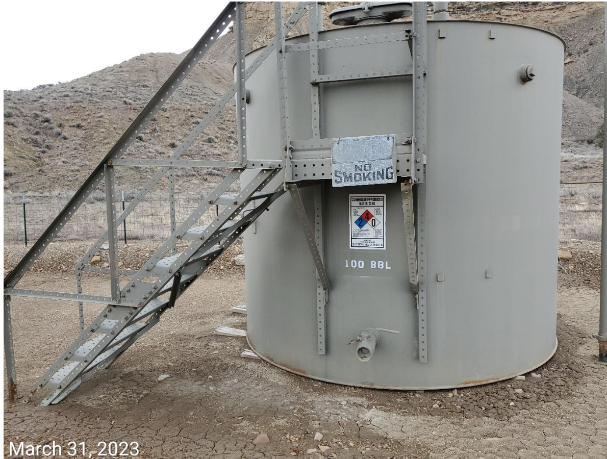
Photo 5: Tank label/signage missing required information per Rule 605.h
