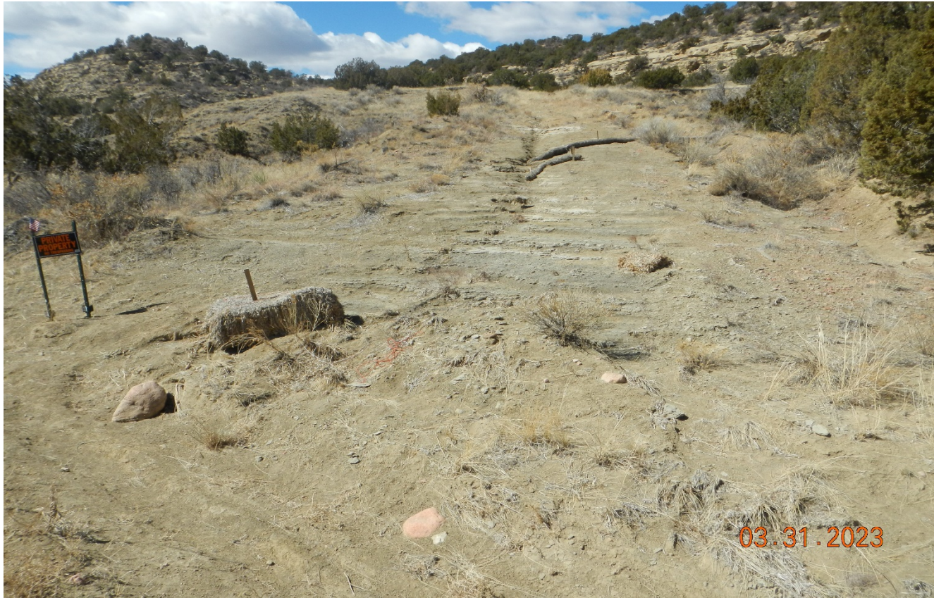
Photo 1. Facing southwest toward the former access road. This area is not stabilized with vegetation and there is erosion has occurred. It appears topsoil has been scoured off this area of the former road.
