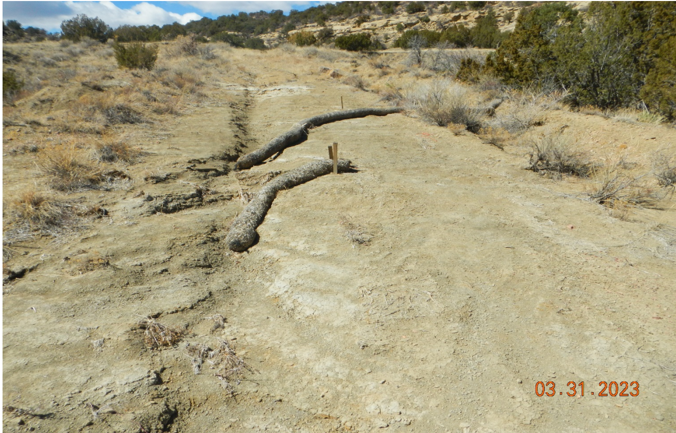
Photo 2. Facing southwest toward the former access road. There were temporary erosion controls installed which have washed out. This area of the access road needs to be reclaimed and stabilized for long term stabilization.
