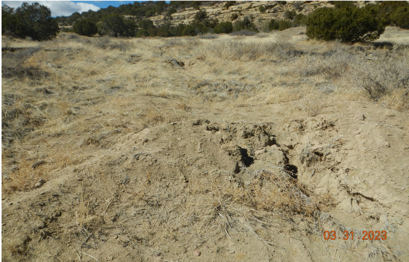
Photo 5. Facing southwest along the access road. It appears soil piles were placed along the road to slow stormwater however they have since eroded and washed out.
