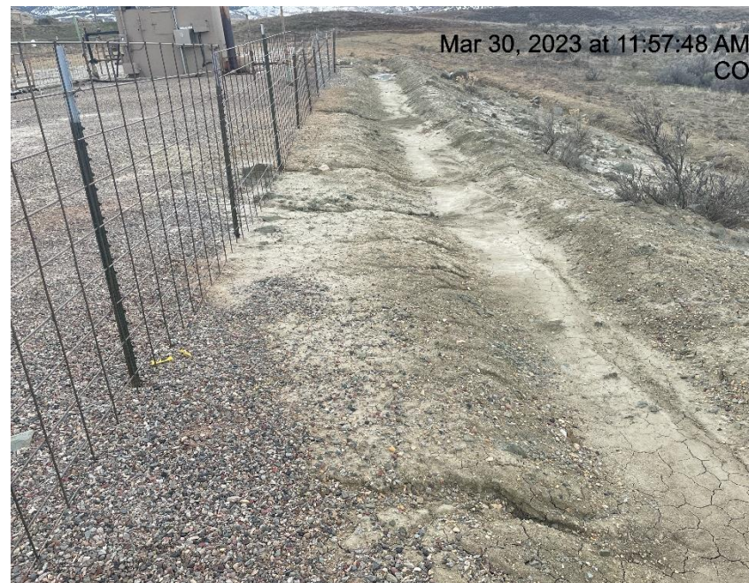
Photo # 3739 Rill erosion & transport of sediment (NW area of location near production tank containment)
