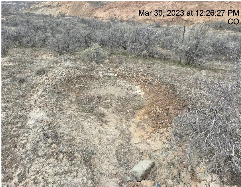
Photo # 3791 Sediment trap needs maintenance (North side of spur road approximately 150-200 yards from entrance to location)
