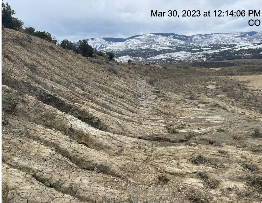
Photo # 3764 Lack of stabilization/Rill & Gully erosion/transport of sediment onto location/insufficient run on controls/BMP's (East side of location on slope)
