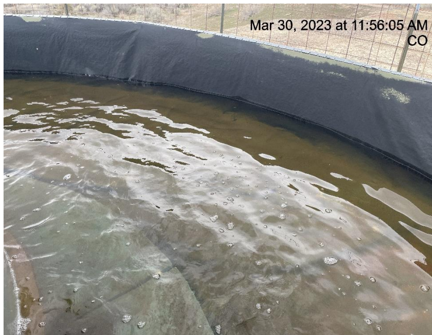
Photo # 3738 Containment capacity inadequate
