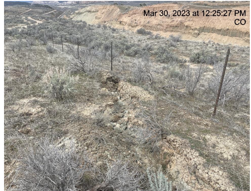
Photo # 3788 Ditch coming out sediment trap/insufficient run off controls/BMP's/erosion & transport of sediment
