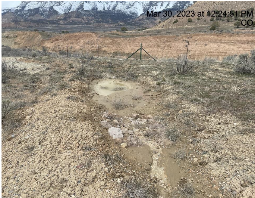
Photo # 3785 Sediment trap needs maintenance (North side of spur road approximately 60 yards from location)
