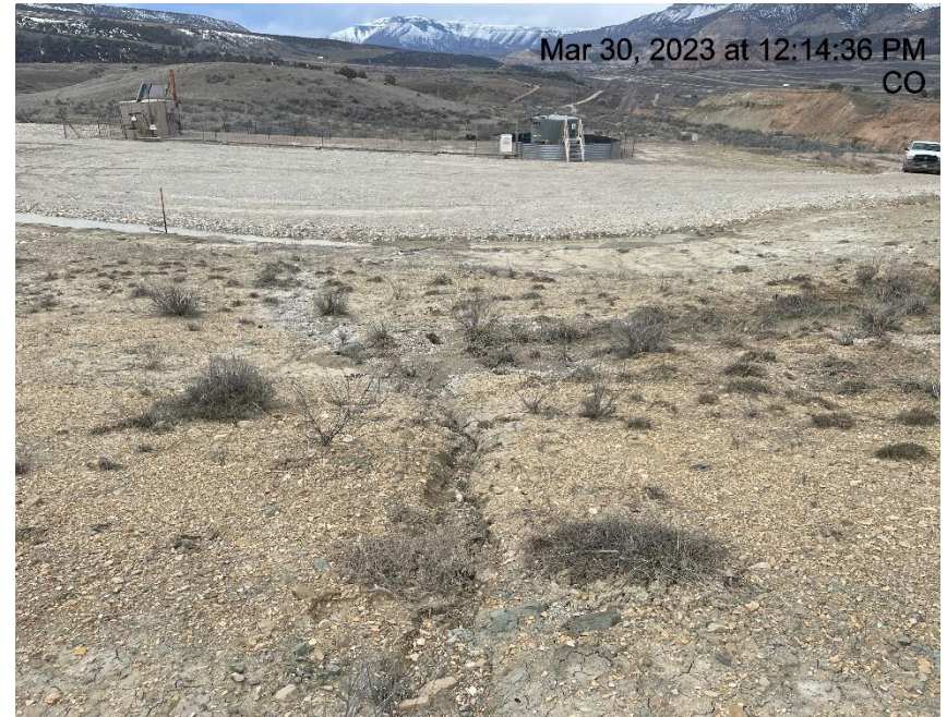
Photo # 3767 Rill erosion (NE area of location)
