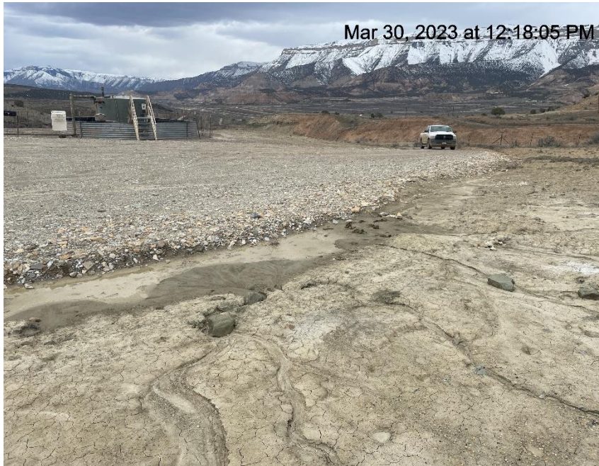
Photo # 3778 Rill erosion (NE area of location)
