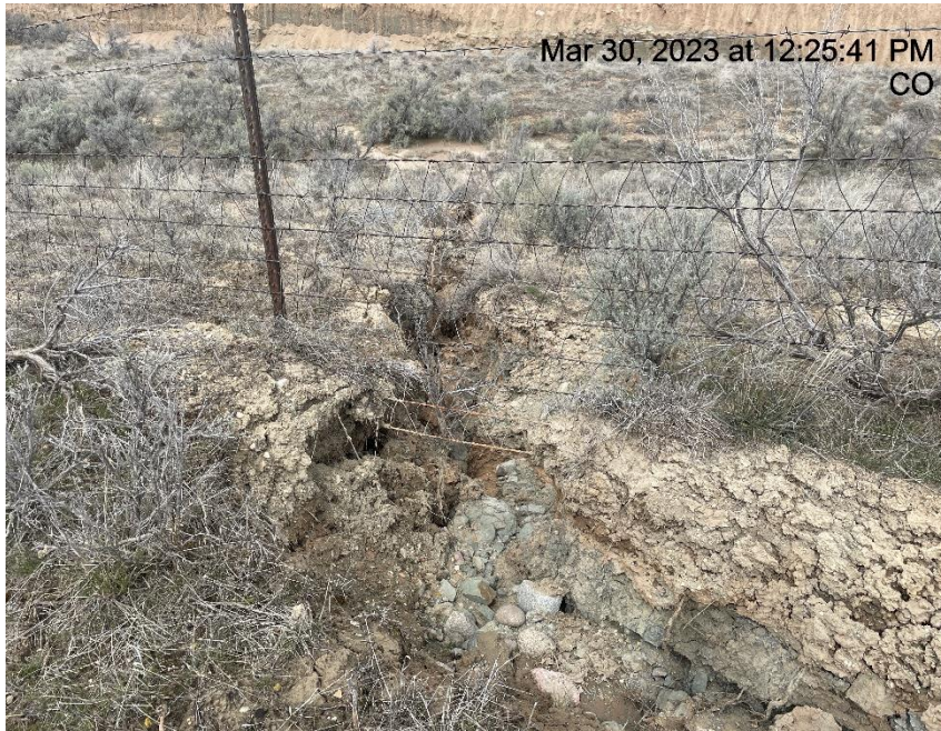
Photo # 3789 Ditch coming out sediment trap/insufficient run off controls/BMP's/erosion & transport of sediment
