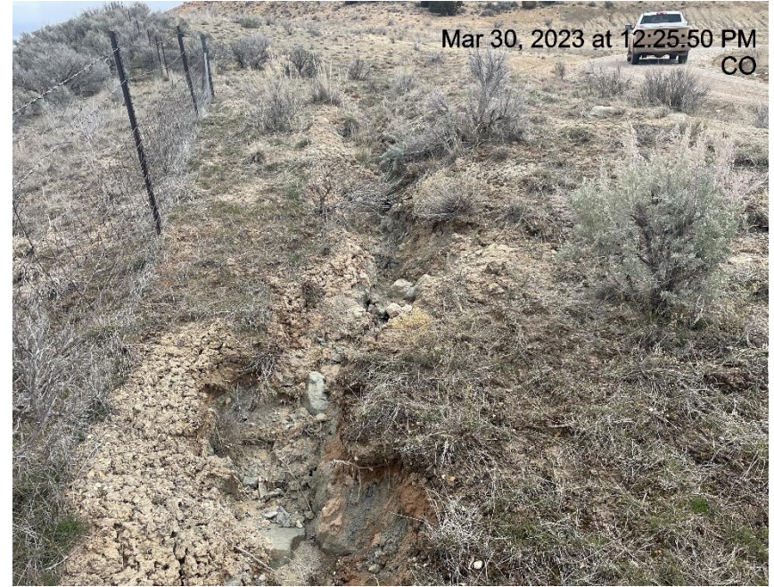
Photo # 3790 Ditch coming out sediment trap/insufficient run off controls/BMP's/erosion & transport of sediment
