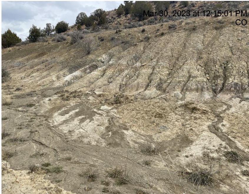
Photo # 3766 Lack of stabilization/Rill & Gully erosion/transport of sediment onto location/insufficient run on controls/BMP's (East side of location on slope)
