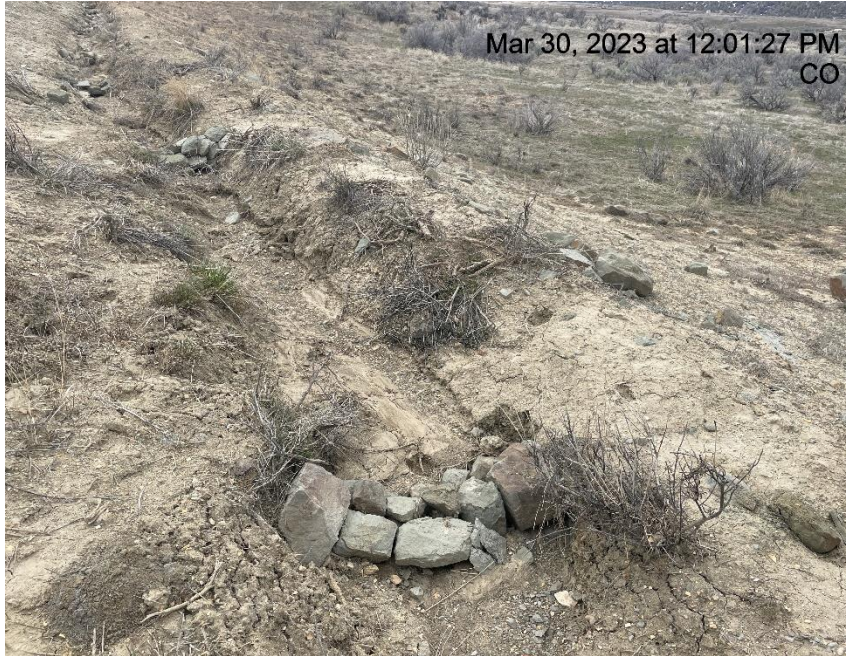
Photo # 3750 Check dam needs maintenance (NW area near sediment trap)
