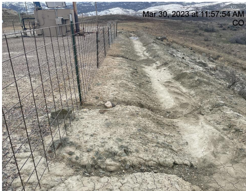
Photo # 3740 Rill erosion & transport of sediment (NW area of location near production tank & containment)
