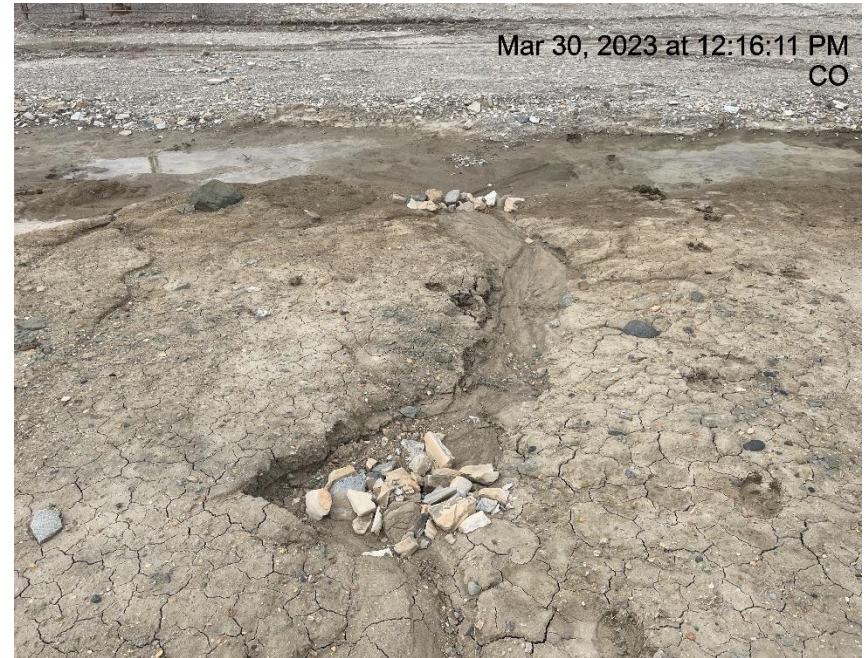
Photo # 3770 Check dam needs maintenance (NE area of location)
