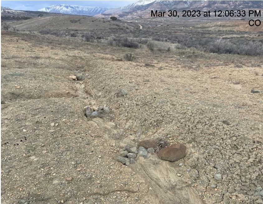
Photo # 3760 Check dam needs maintenance (SW area of location)
