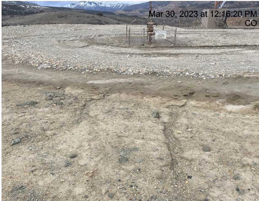
Photo # 3771 Rill erosion (SE area of location)
