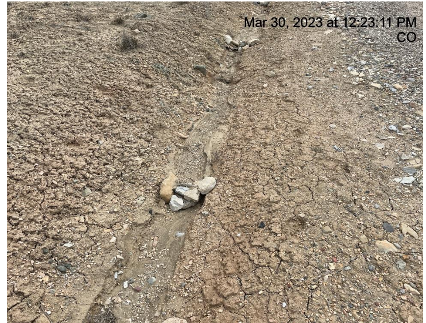
Photo # 3782 Check dam needs maintenance (NE area of location)
