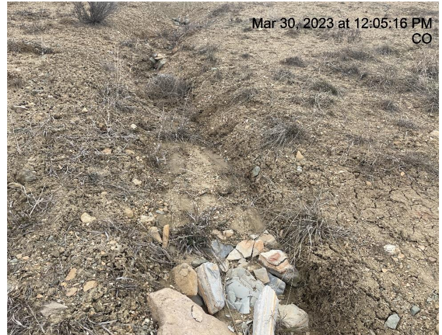
Photo # 3758 Check dam needs maintenance (SW area of location)
