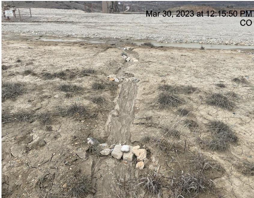
Photo # 3769 Check dam needs maintenance (NE area of location)
