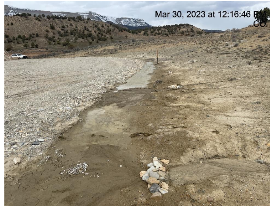
Photo # 3773 Check dam & ditch need maintenance (East side of location)
