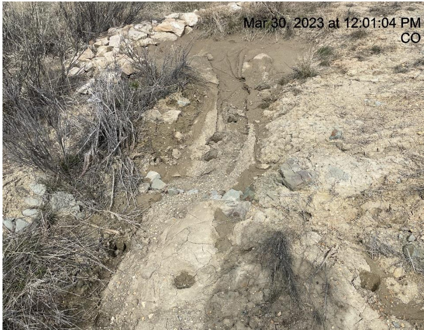
Photo # 3748 Sediment Trap needs maintenance (NW area of location)
