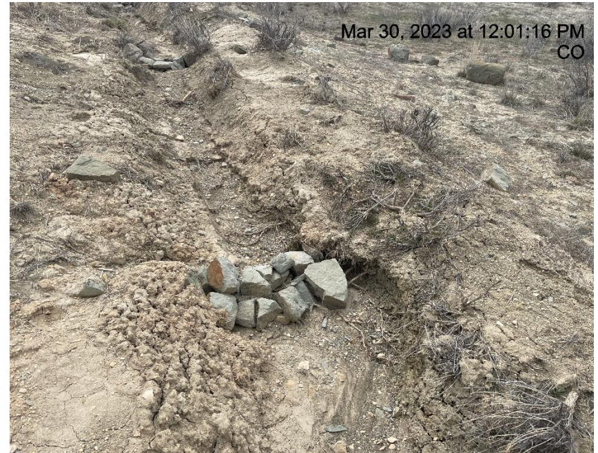
Photo # 3749 Check dam needs maintenance (NW area near sediment trap)
