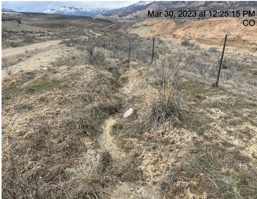
Photo # 3787 Ditch coming out sediment trap/insufficient run off controls/BMP's/erosion & transport of sediment
