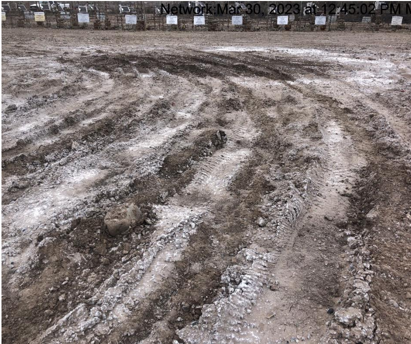
Photo #9440 Location lacks stabilization.
