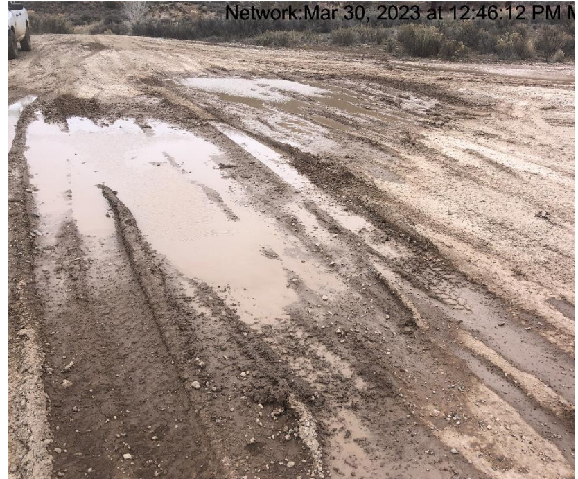
Photo #9446 Location lacks stabilization.
