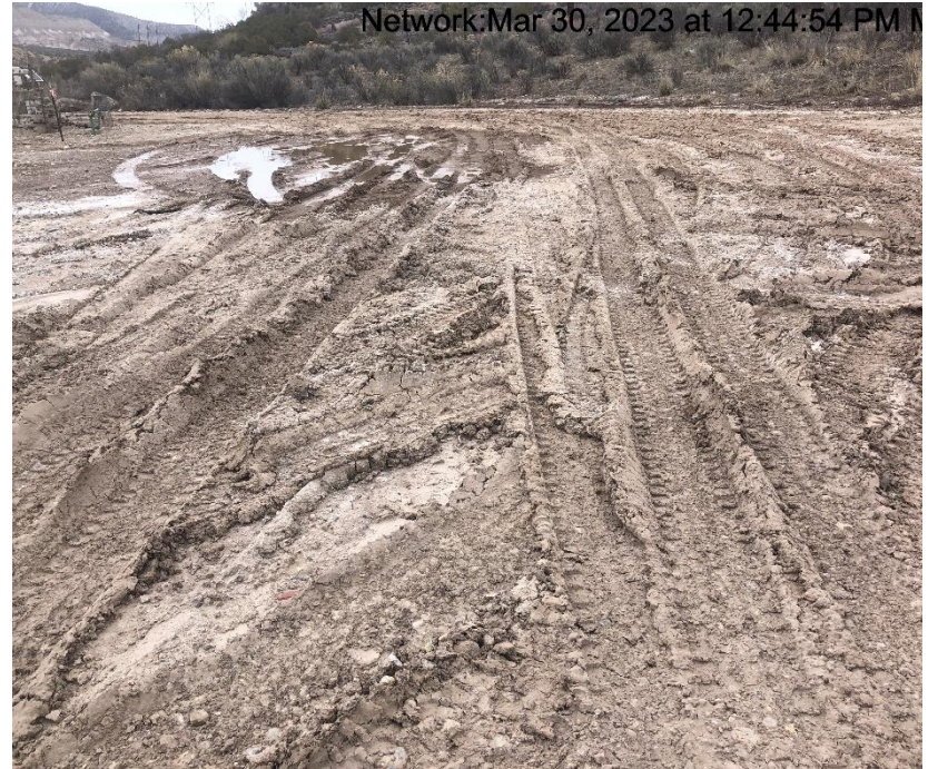
Photo #9437 Location lacks stabilization.
