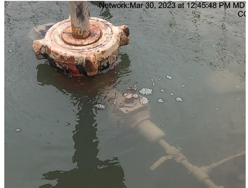
Photo #9444 Well W 15-5 wellhead leaking.
