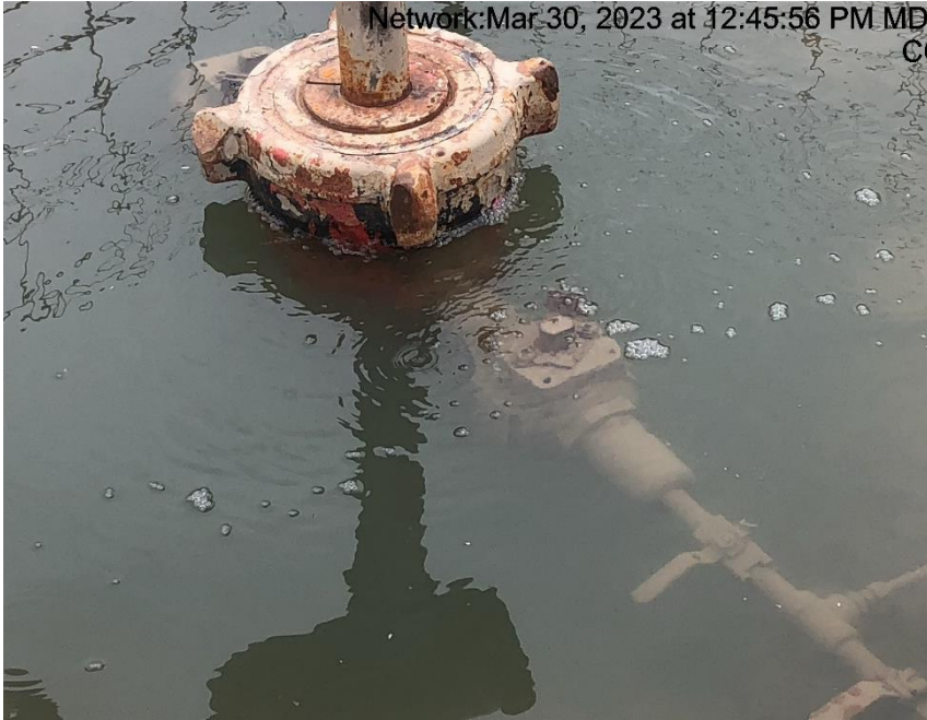
Photo #9445 Well W 15-5 wellhead leaking
