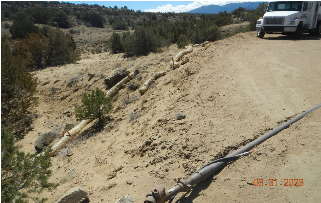
Photo 21. Facing southeast along the fill slope of the pad. There are wattles installed however they are not properly installed per good engineering practice. Wattles are not properly positioned, trenched, or staked down.
