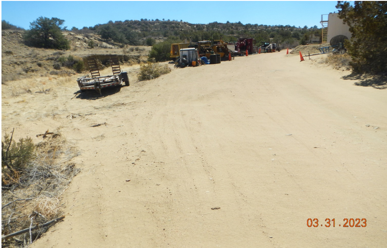
Photo 2. Facing southeast long the access road at the tank battery site. The trailer is being parked off the access road creating additional disturbance. The loose soils along the road are susceptible to erosion.
