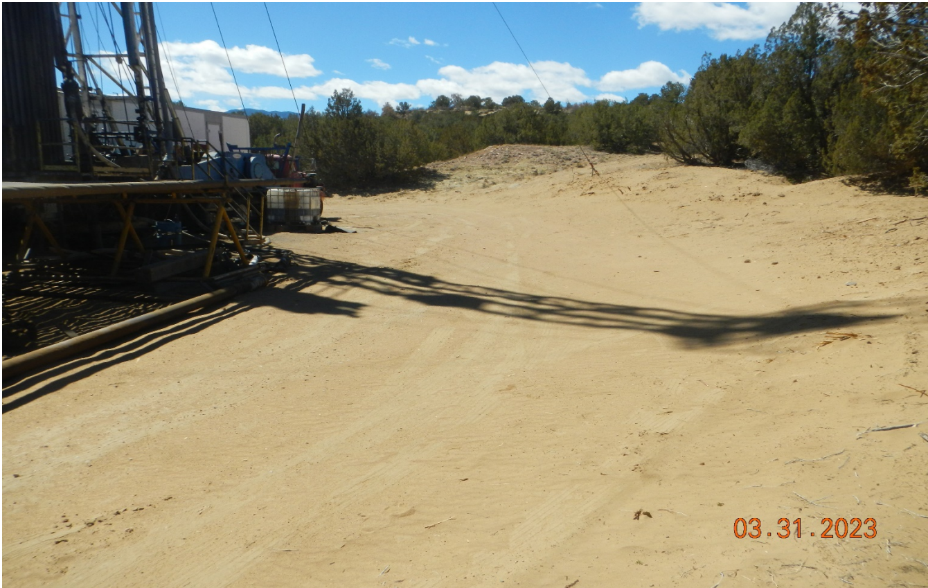
Photo 27. Facing southwest at the location. There are no stormwater run-on controls along the west side of the location.
