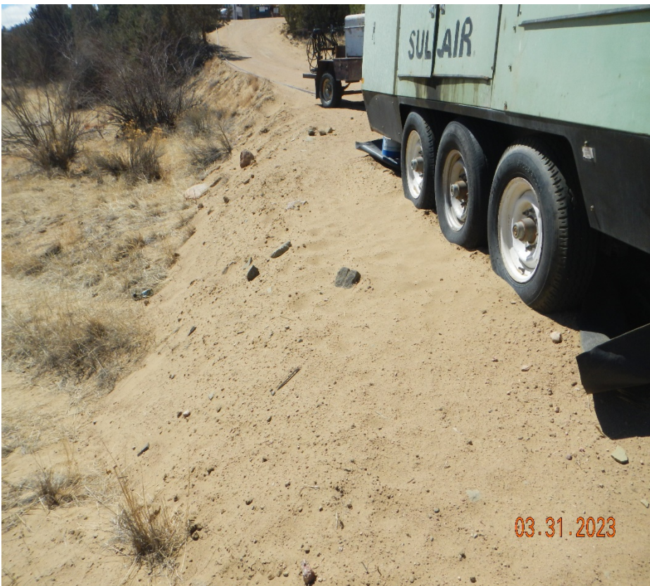
Photo 11. Facing south at the east side of the tank battery where equipment is being stored. There are no stormwater controls to prevent erosion of loose soils.
