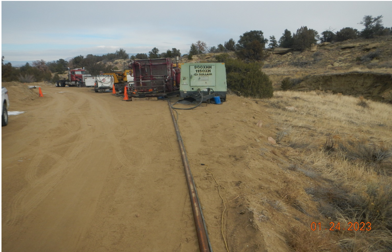
Photo 15. Facing north at the tank battery site where equipment is being stored. There are no perimeter stormwater controls down gradient toward the stream drainage at right side of photo which previous inspection also cited.
