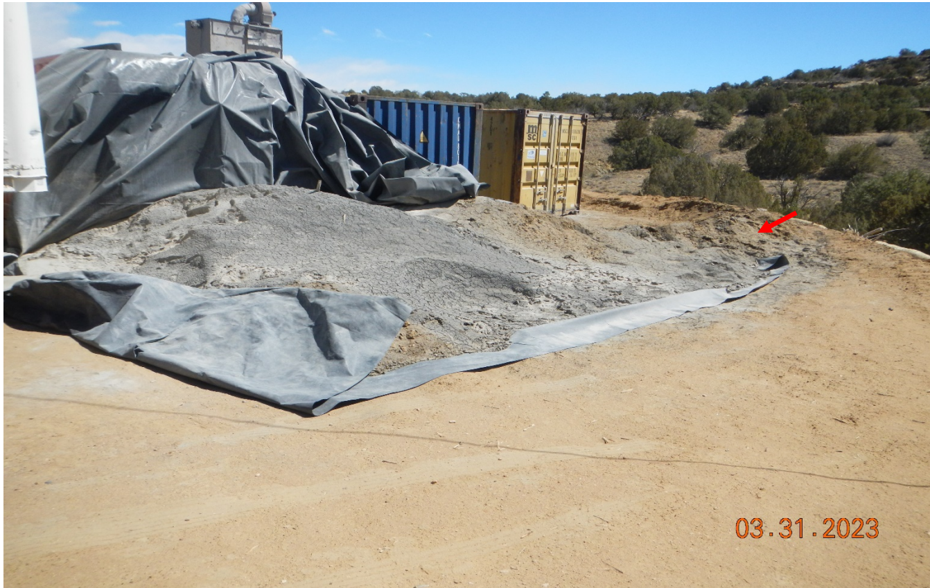
Photo 25. There is drill cuttings on the surface not properly stored and contained. The plastic liner does not contain the drill cutting from stormwater run-off and part of the cuttings at red arrow is not even off the edge of the liner.
