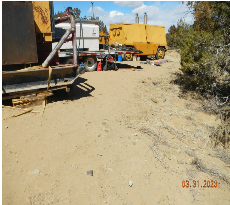
Photo 12. Facing north at the east side of the tank battery where equipment is being stored. There are no stormwater controls to prevent erosion of loose soils.
