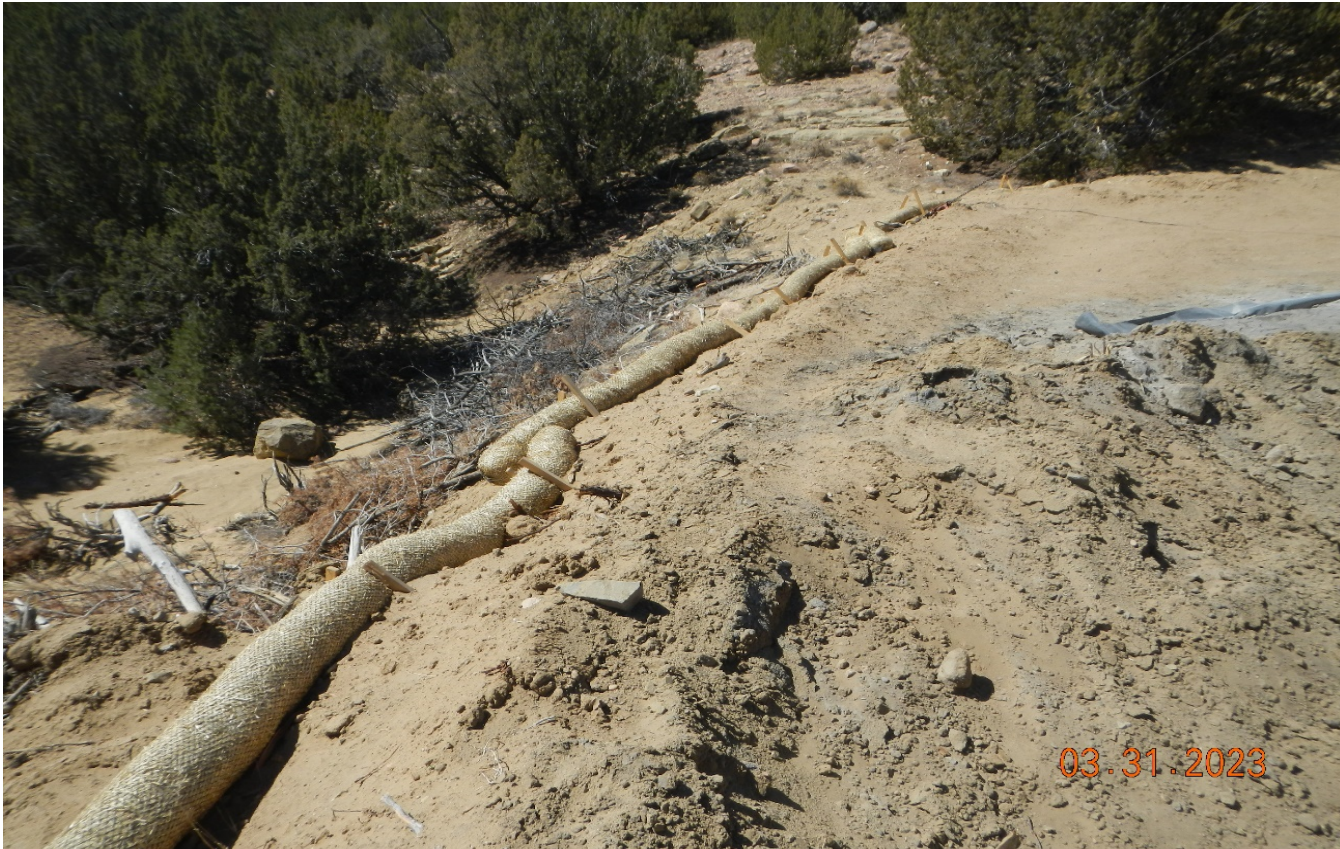
Photo 22. The wattle installed at the southern perimeter should have been position at the bottom of the slope to contain all loose soils that were pushed out and disturbed. BMP's need to be properly installed per good engineering practice.
