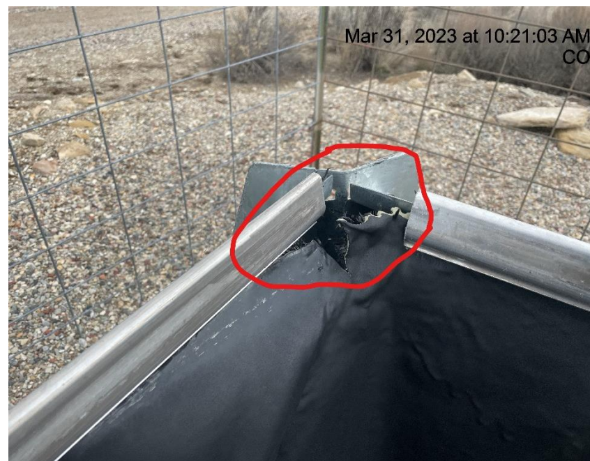
Photo # 3937 Containment liner needs maintenance
