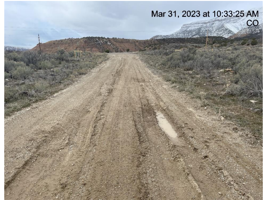
Photo # 3948 Lack of stabilization/Insufficient tracking BMP's
