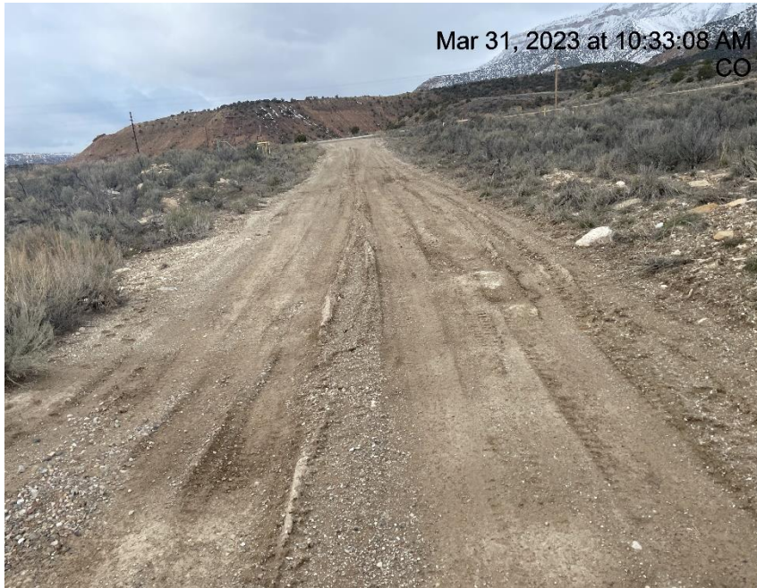
Photo # 3947 Lack of stabilization/Insufficient tracking BMP's
