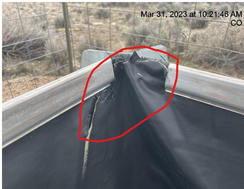
Photo # 3940 Containment liner needs maintenance
