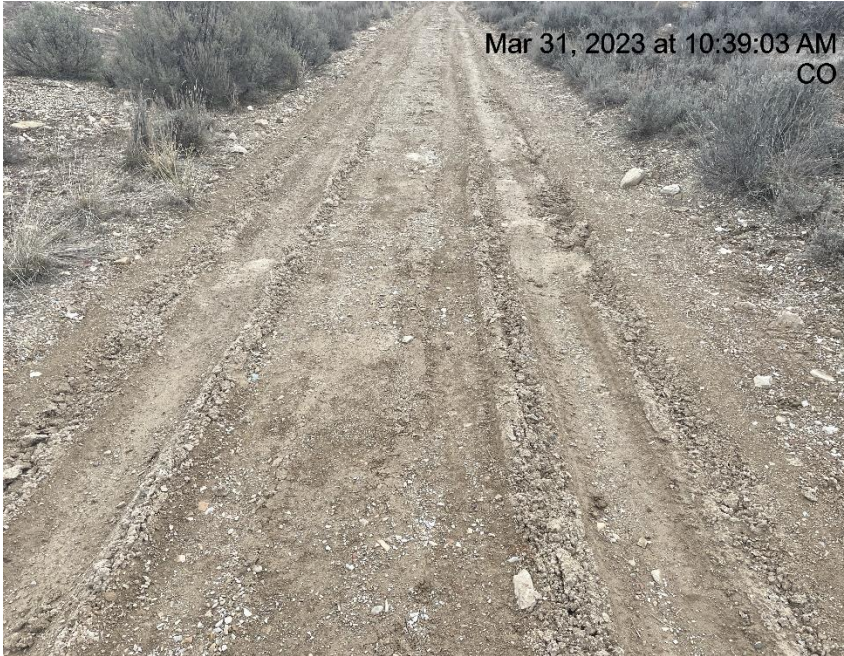
Photo # 3955 Lack of stabilization/Insufficient tracking BMP's
