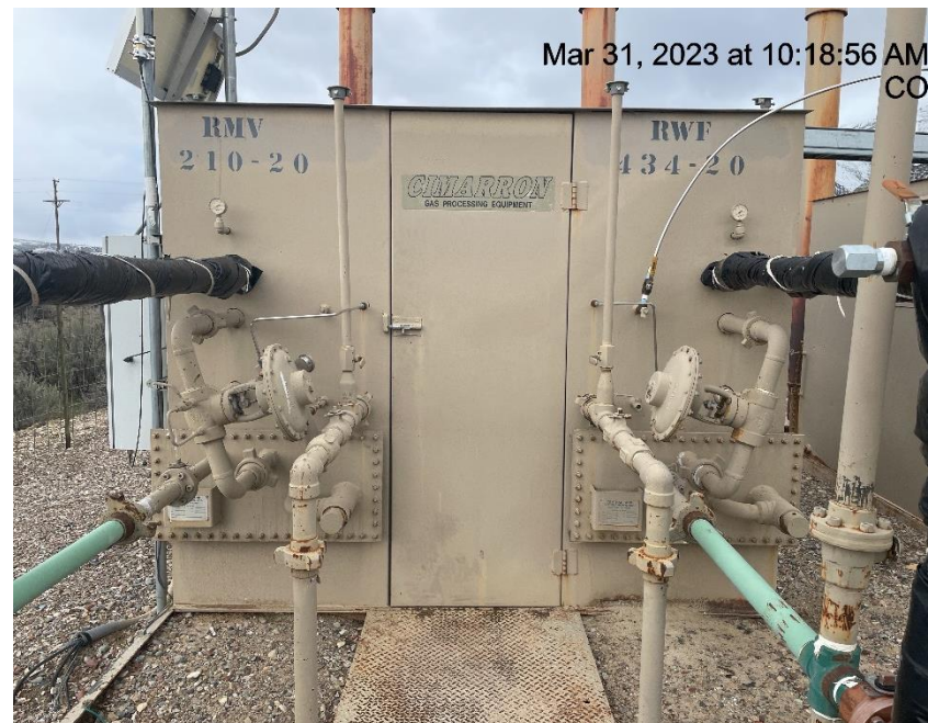
Photo # 3933 Meter calibration info not conspicuously posted
