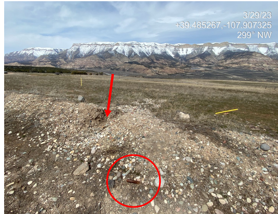
Photo 6. Photo shows an unmarked anchors to the north of the wells. Photo also shows where a perimeter stormwater berm has been blown out.
