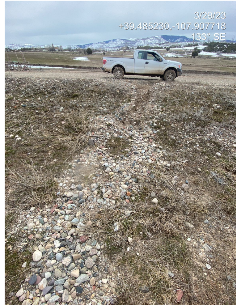
Photo 7. Photos taken to the north of the wells show multiple areas where the perimeter stormwater berm has been blown out.
