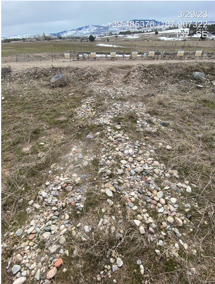
Photo 7. Photos taken to the north of the wells show multiple areas where the perimeter stormwater berm has been blown out.
