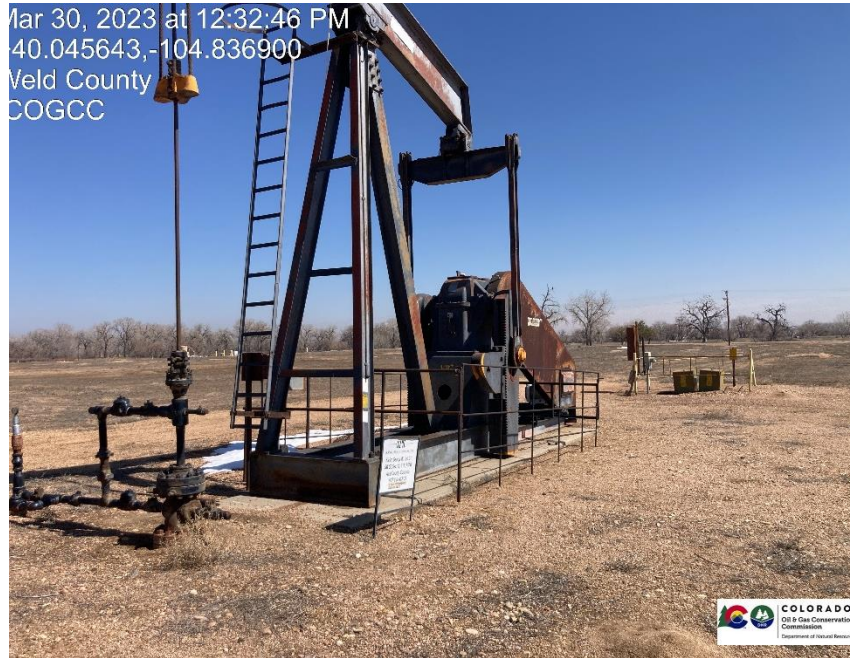
Pic 1 wellhead / pumpjack / Electric equip.
