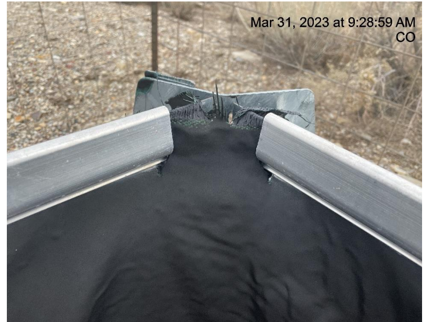
Photo # 3897 Containment liner needs maintenance
