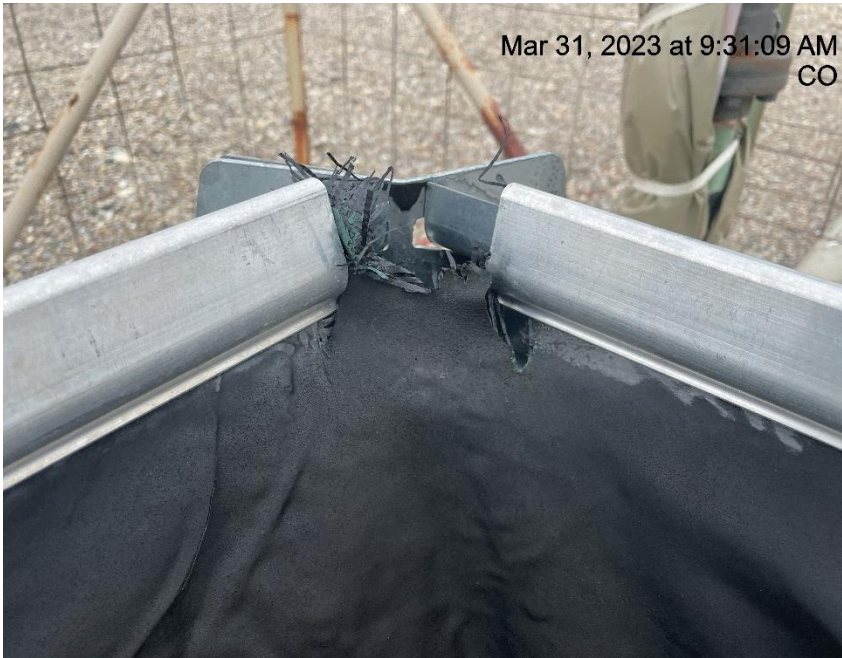
Photo # 3901 Containment liner needs maintenance
