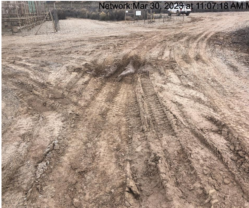
Photo #9417 Location lacks stabilization.
