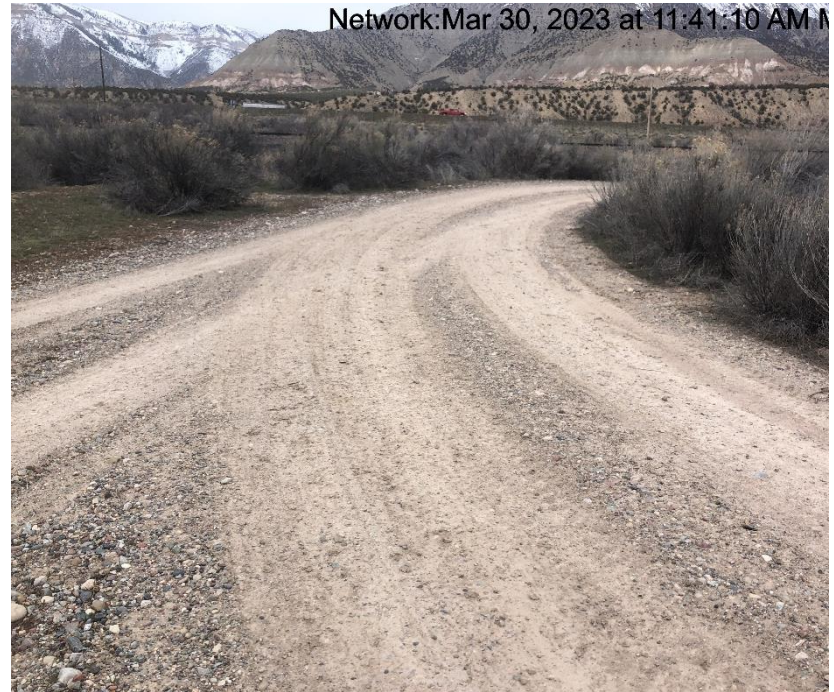
Photo #9425 Insufficient tracking BMP at entrance to location.
