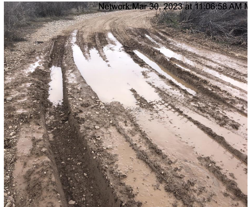
Photo #9416 Location lacks stabilization.
