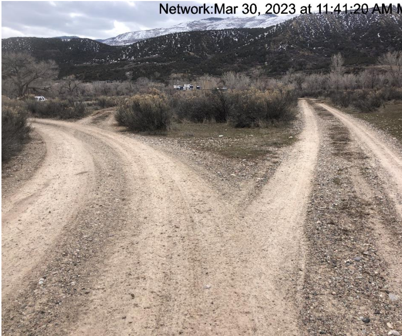
Photo #9426 Insufficient tracking BMP at entrance to location.
