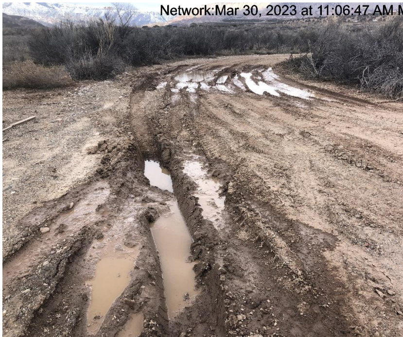
Photo #9415 Location lacks stabilization.
