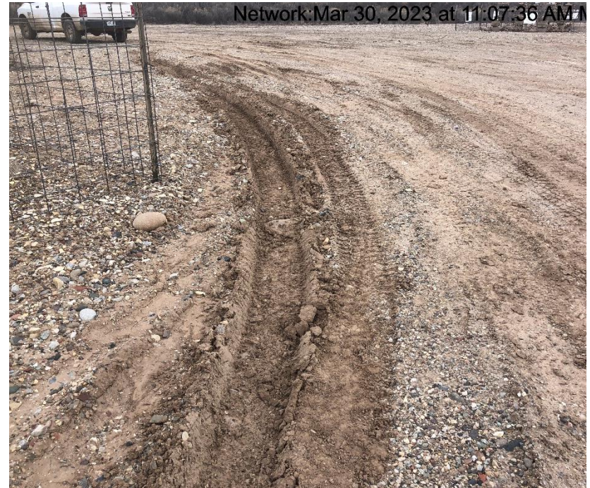
Photo #9418 location lacks stabilization.
