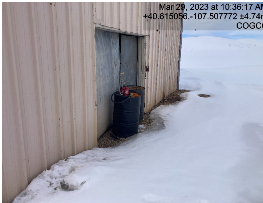
Drums unlabeled and not contained
