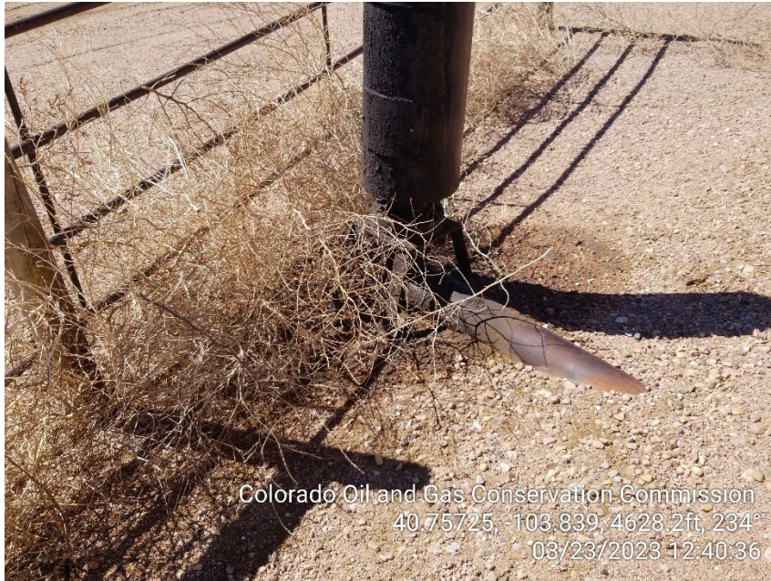
Photo 7 – Stained Soil at Exhaust
