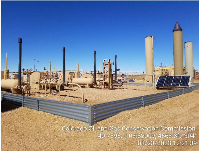
Photo 7 – Separators and ECDs
