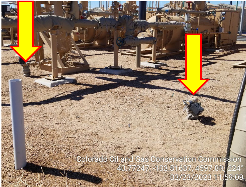
Photo 7 – Unmarked Risers at Headers
