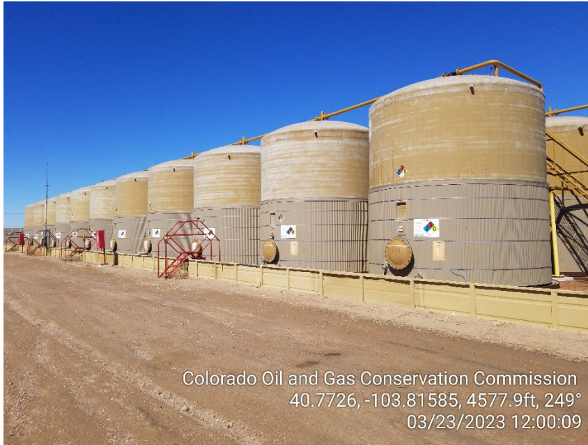
Photo 9 – Produced Water Tanks
