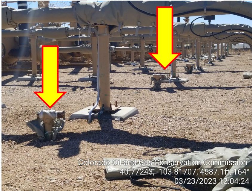
Photo 19 – Unmarked Risers at Headers
