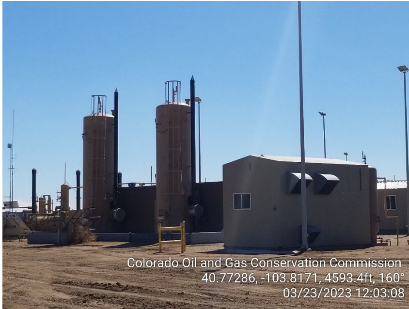
Photo 17 – Heater Treater and Instrumental Air Unit
