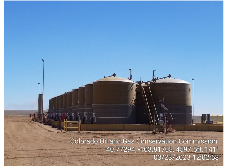
Photo 16 – Produced Water Tank
