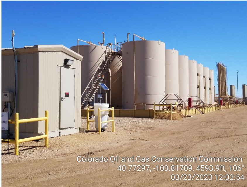
Photo 15 – LACT and Tank Battery
