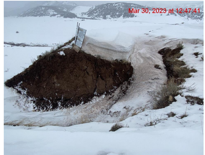
Cut Slope Erosion/Run-off – Photo #01773
