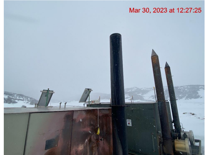
Missing Wildlife Protection – Photo #01765
