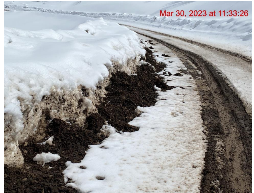
Transport of Sediment/Lack of Stabilization – Photo #01733
