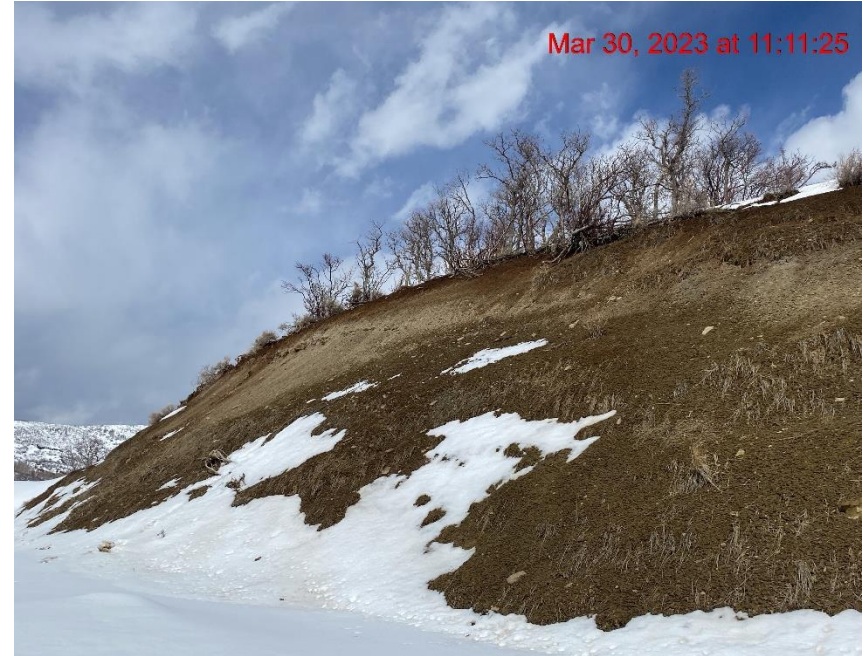
Cut Slope Erosion/Run-On to Location – Photo #01729
