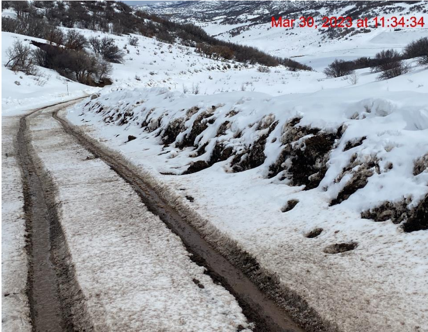
Transport of Sediment/Lack of Stabilization – Photo #01734
