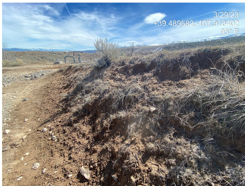
Photo 9. Photos show pedestal erosion throughout the cut slope at the south of the location.
