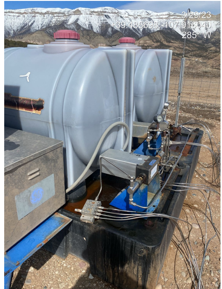
Photo 4. Photo shows a leaky chemical injection unit located at the wells.
