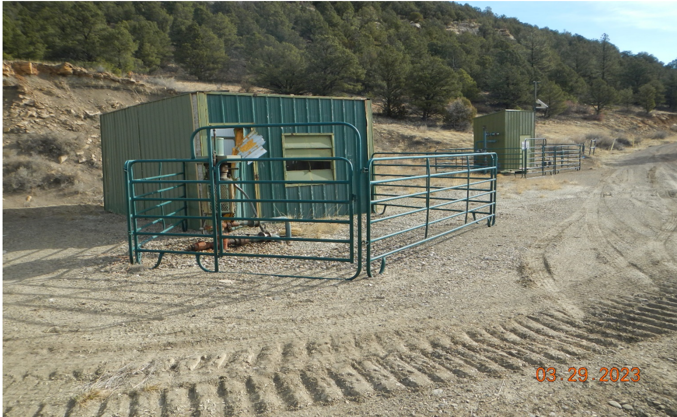
Photo 2. Panels are installed around wellhead.
