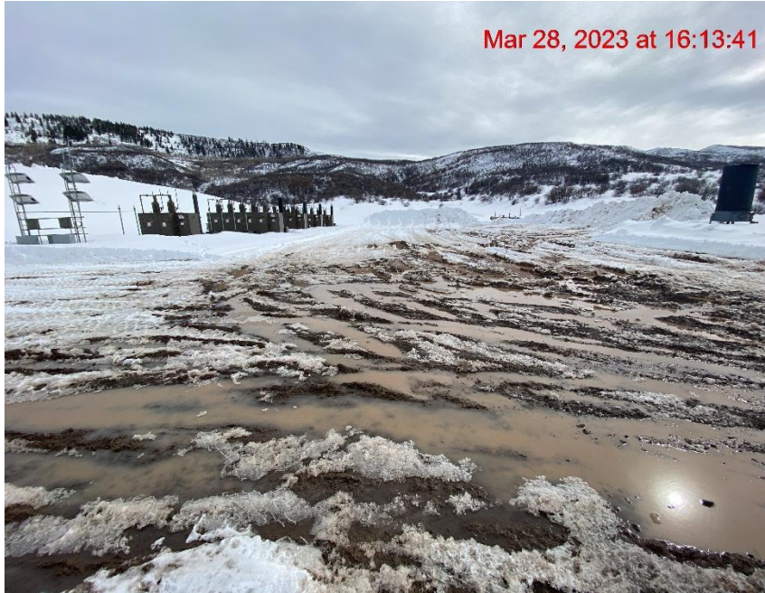
Lack of Stabilization – Photo #01707
