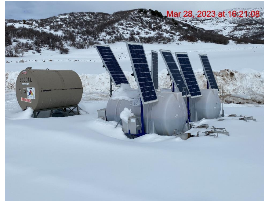
Chemical Tanks/Inadequate Secondary Containment – Photo #01717
