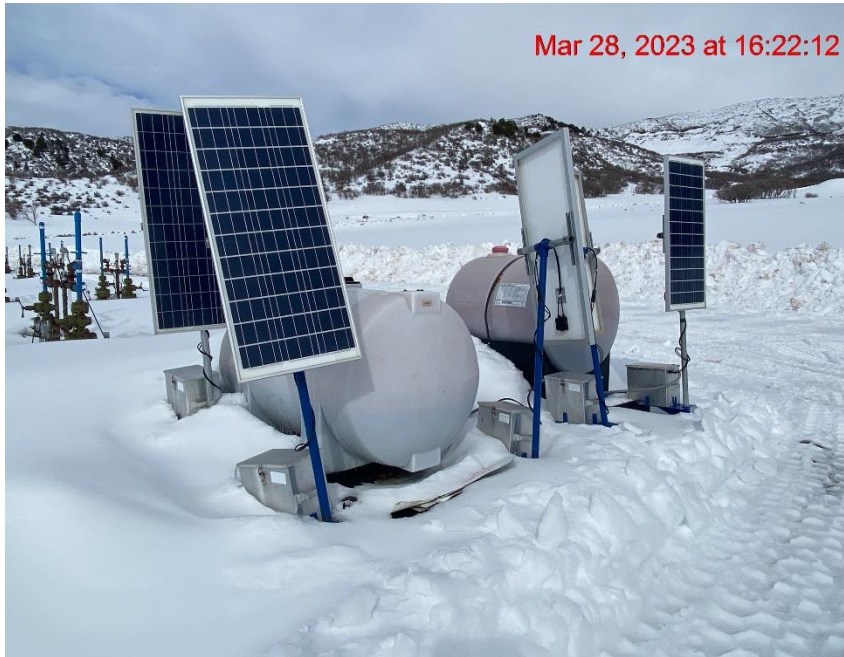
Chemical Tanks/Inadequate Secondary Containment – Photo #01718
