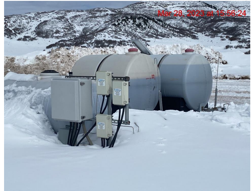
Inadequate Chemical Secondary Containment – Photo #01688
