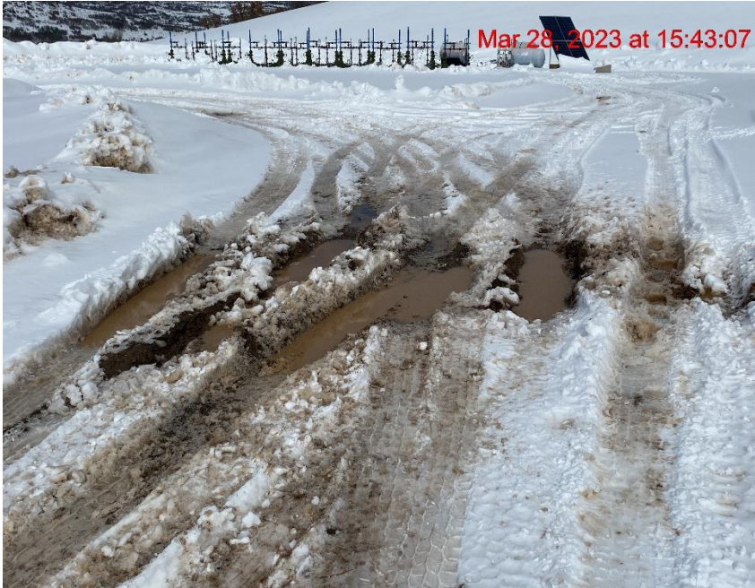
Lack of Stabilization – Photo #01684
