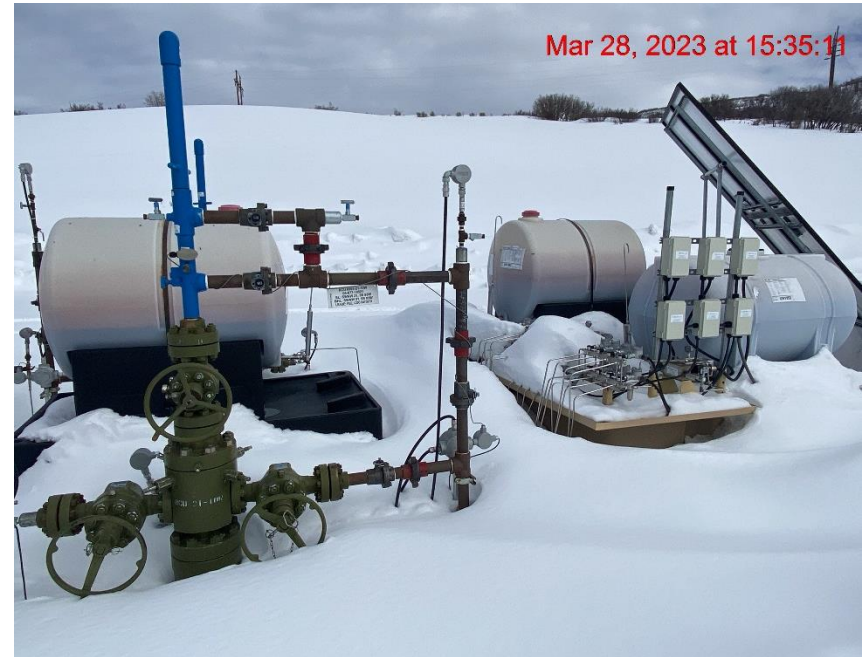
Inadequate Chemical Containment – Photo #01669
