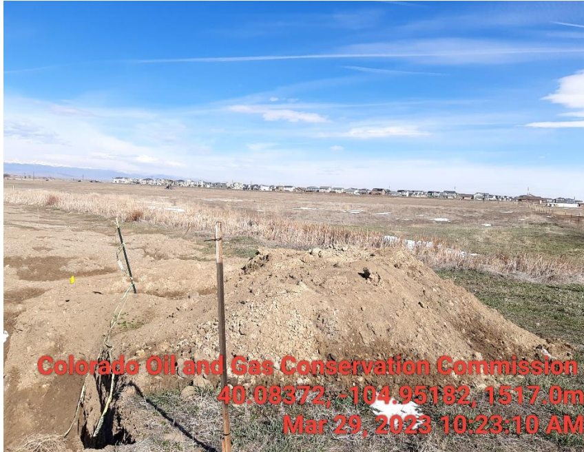
Photo 11 open excavation stock pile material no BMP' in wetland
