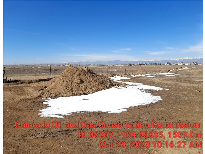
Photo 4 Excavation material not BMP
