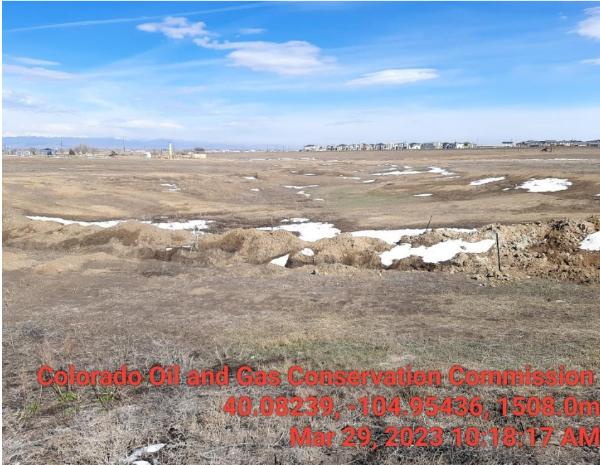
Photo 5 Open excavation looking North no BMP's in creek crossing
