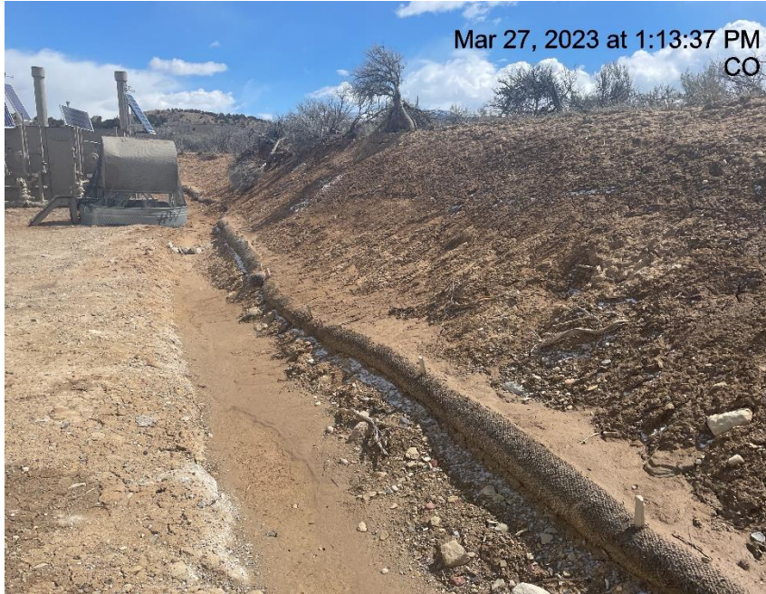
Photo # 3446 Insufficient run on controls/BMP's
