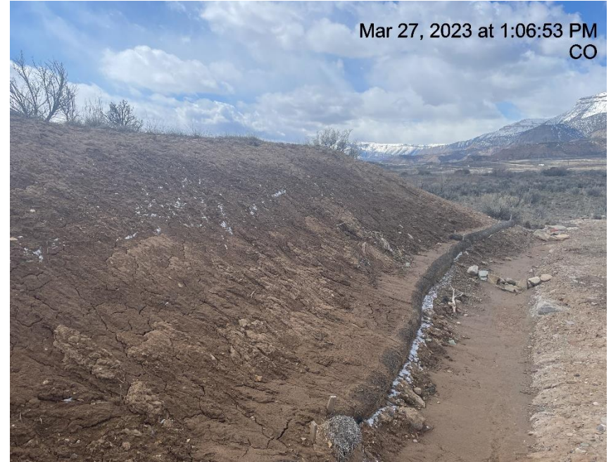
Photo # 3436 Lack of stabilization & erosion of cut slope/ insufficient BMP's & insufficient run on controls/BMP's
