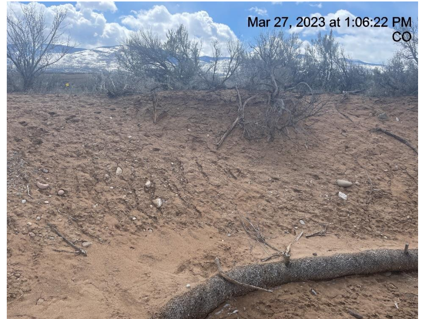
Photo # 3434 Lack of stabilization & erosion of cut slope/ insufficient BMP's
