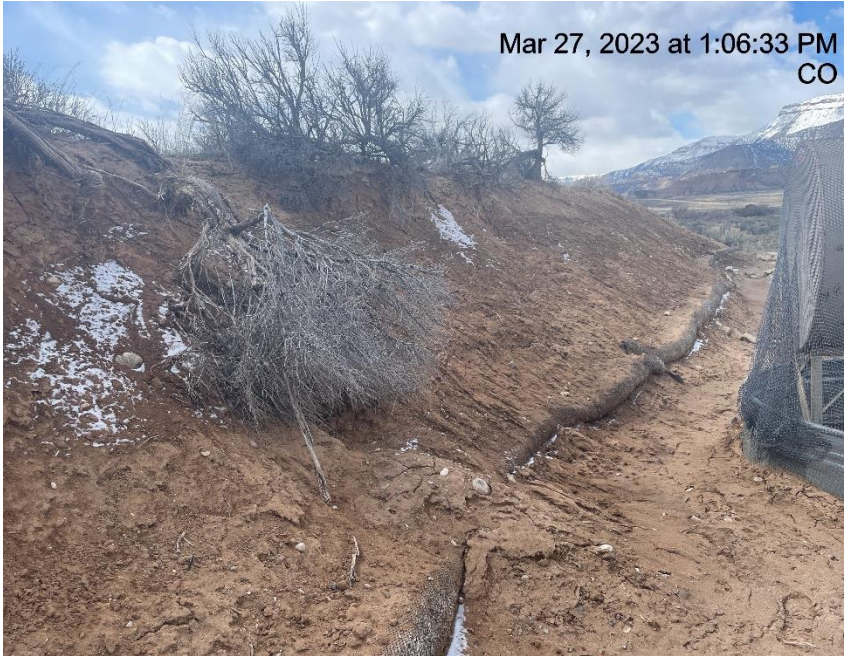
Photo # 3435 Lack of stabilization & erosion of cut slope /insufficient BMP's & insufficient run on controls/BMP's
