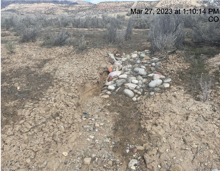
Photo # 3442 Rip Rap needs maintenance (NW area of location across from wellheads)
