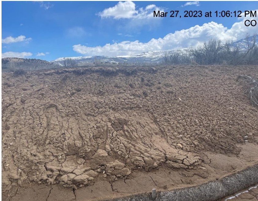
Photo # 3433 Lack of stabilization & erosion of cut slope/ insufficient BMP's
