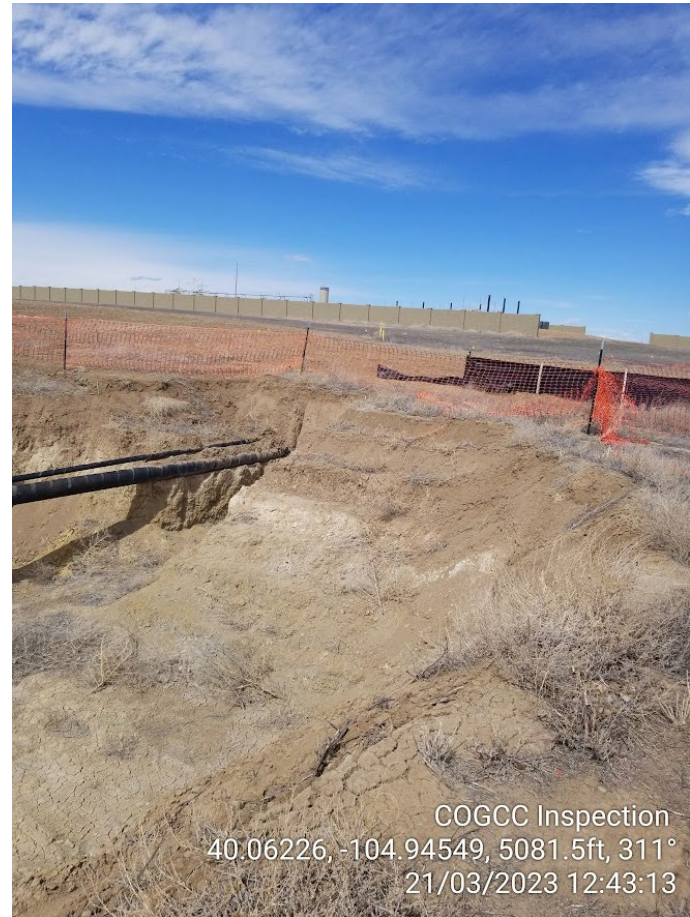
Photo 2 – Excavation- note silt fence failing in background
