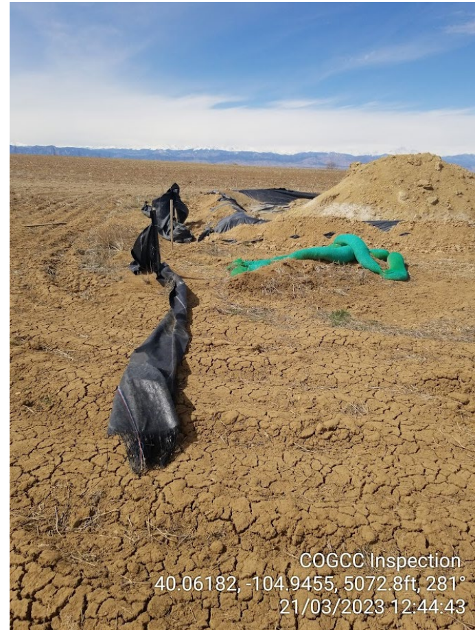
Photo 6 – Failed stormwater BMPs and trash
