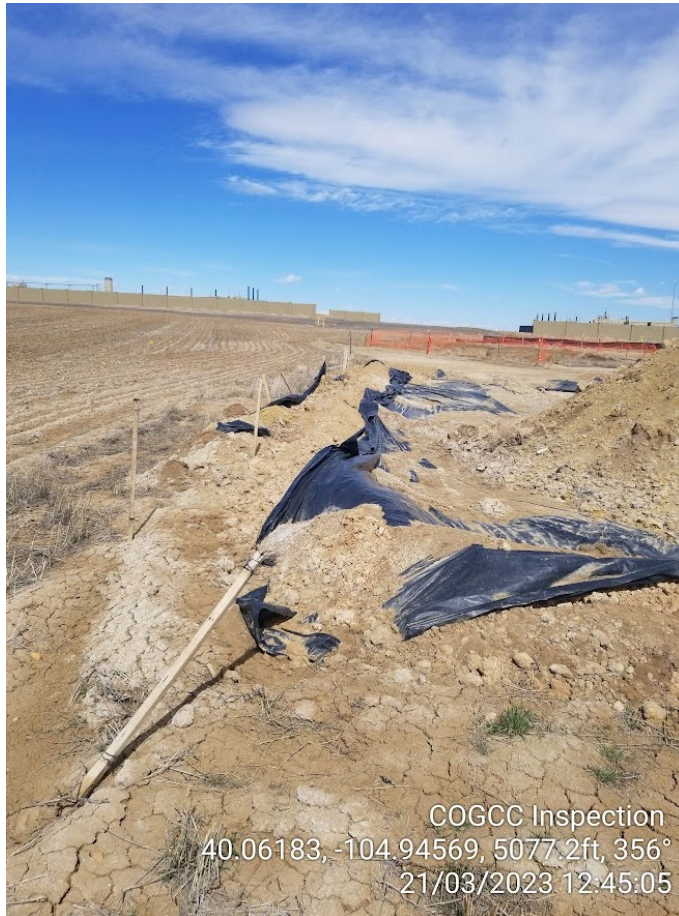
Photo 7 – South Excavation Failed stormwater BMPs and contaminated soils overtopping berm.
