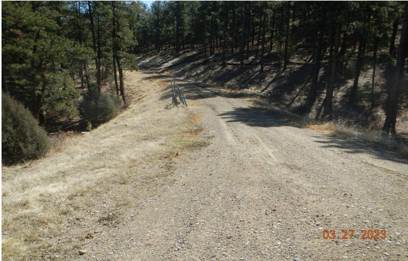
Photo 1. Facing east at beginning of the access road.
