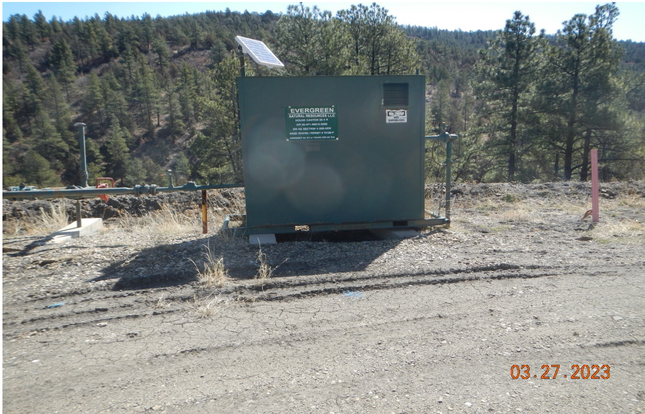
Photo 3. Well sign posted at meter shed.
