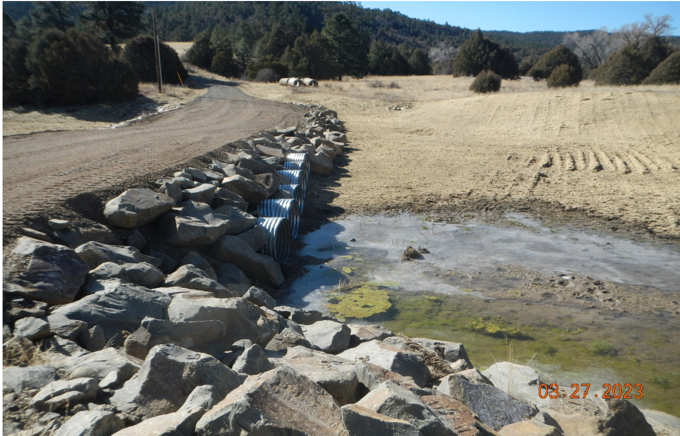
Photo 1. Facing south toward the access road stream crossing. There has been additional culverts installed and the embankment has been armored with rock rip/rap protection. Previous corrective action has been completed.
