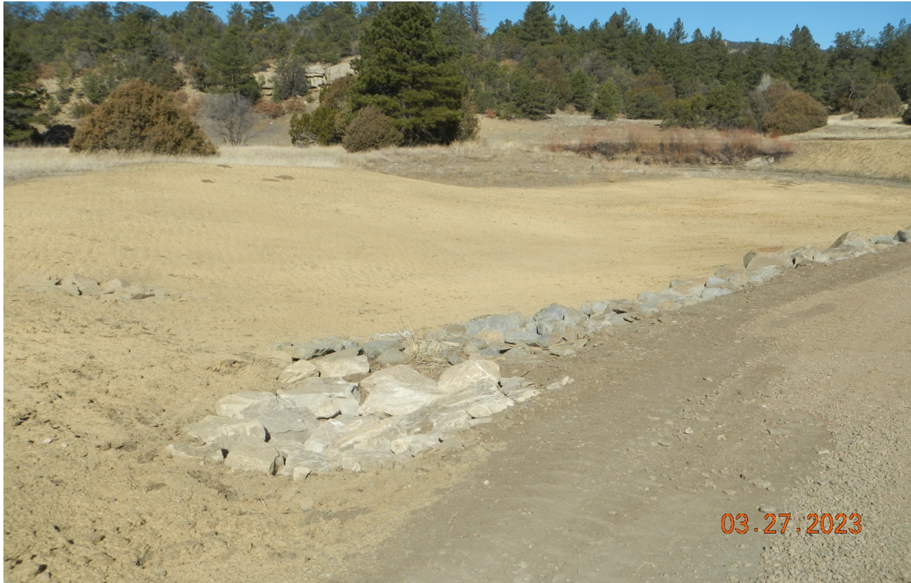
Photo 4. All disturbed areas along the road side have been seeded and stabilized.
