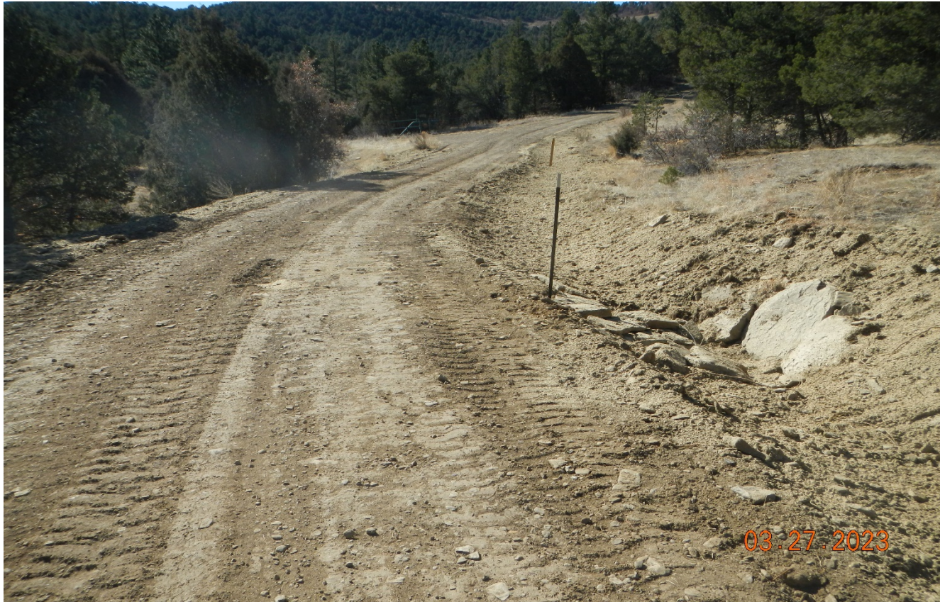
Photo 5. Facing southeast along the access road. The road side has been seeded and stabilized. The culverts are maintained.
