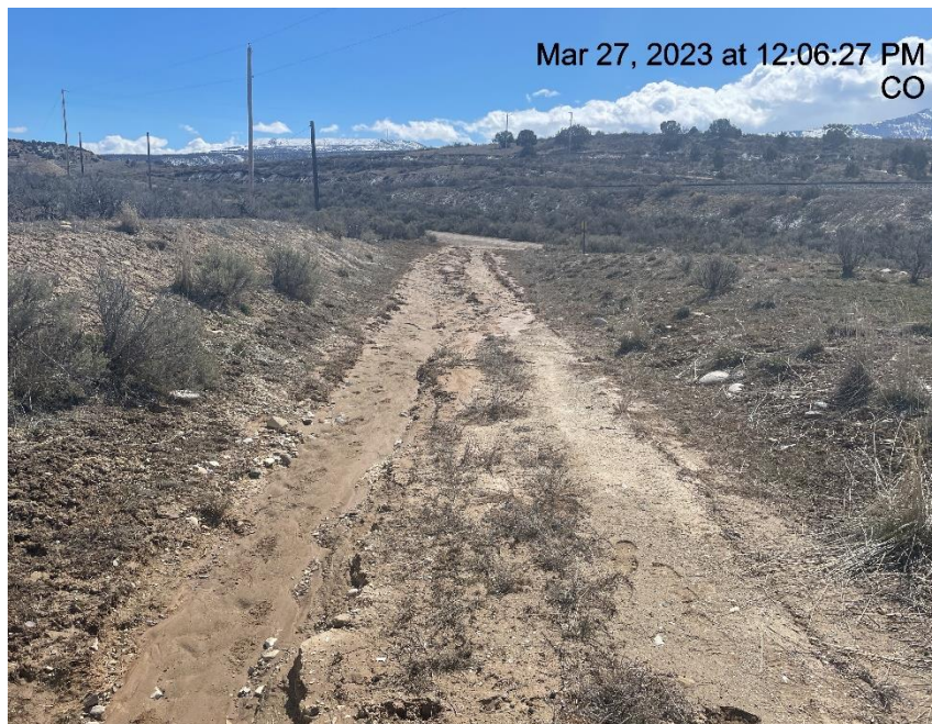
Photo # 3392 Rill erosion & transport of sediment on spur road
