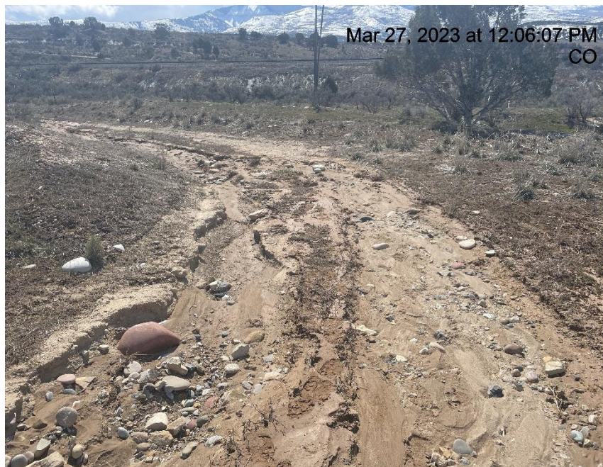
Photo # 3390 Rill erosion & transport of sediment on spur road
