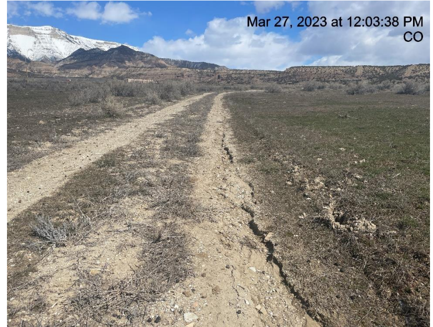
Photo # 3383 Rill erosion on spur road
