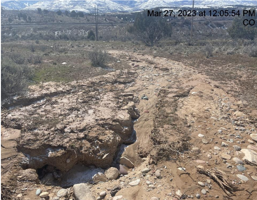
Photo # 3388 Gully/Rill erosion/Transport of sediment on spur road/road degradation
