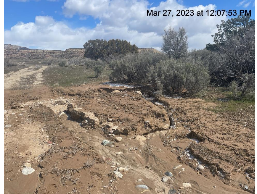
Photo # 3389 Gully/Rill erosion/Transport of sediment on spur road/road degradation
