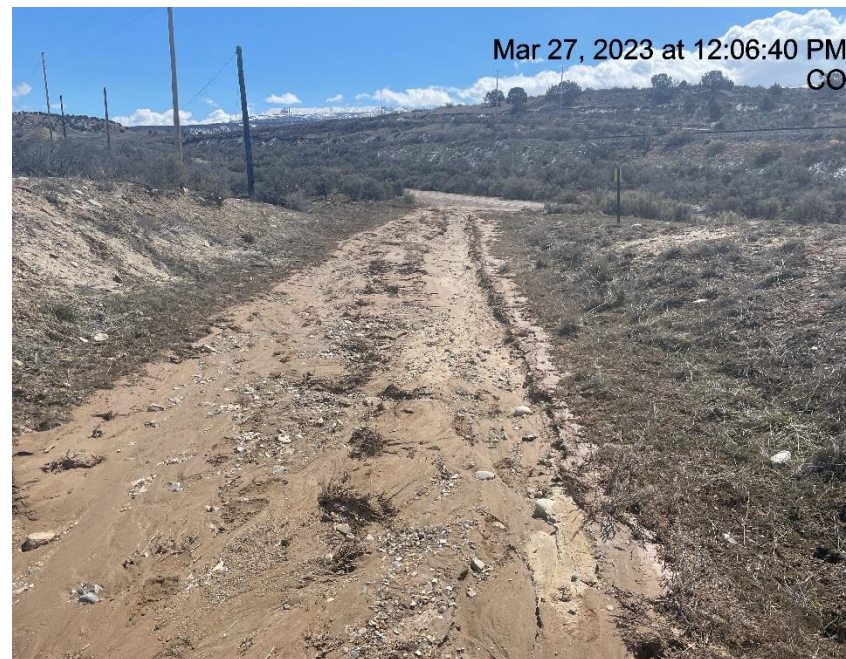
Photo # 3393 Rill erosion & transport of sediment on spur road
