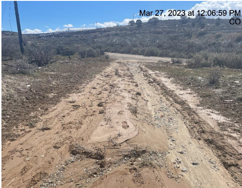
Photo # 3394 Rill erosion & transport of sediment on spur road
