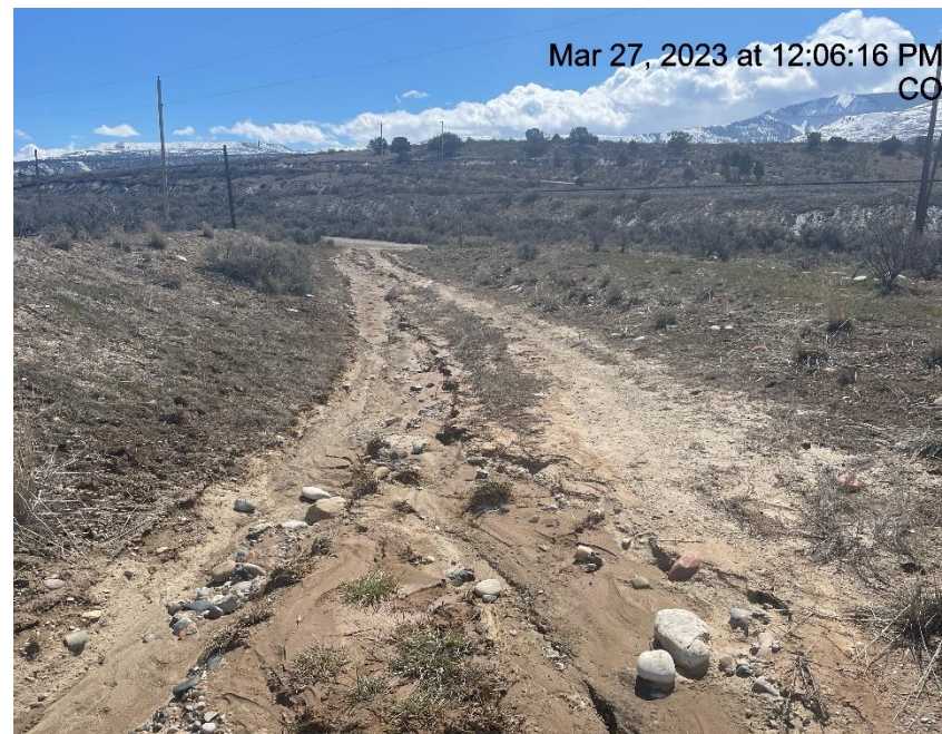
Photo # 3391 Rill erosion & transport of sediment on spur road
