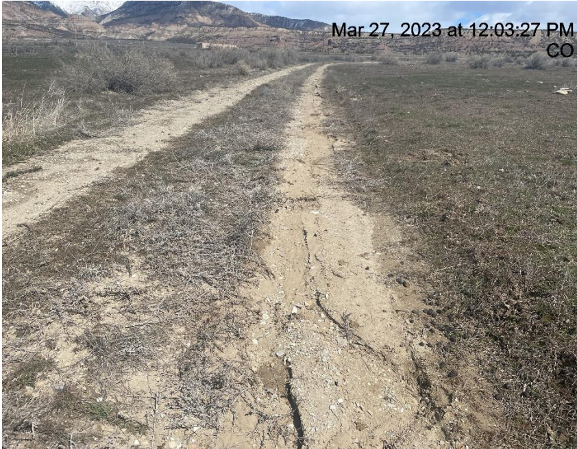
Photo # 3382 Rill erosion on spur road
