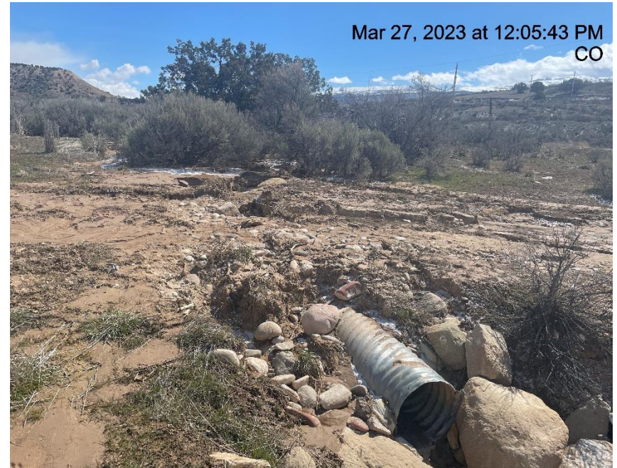
Photo # 3387 Culvert needs maintenance/Insufficient run on BMP's
