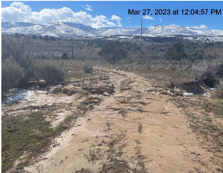
Photo # 3384 Road degradation/transport of sediment
