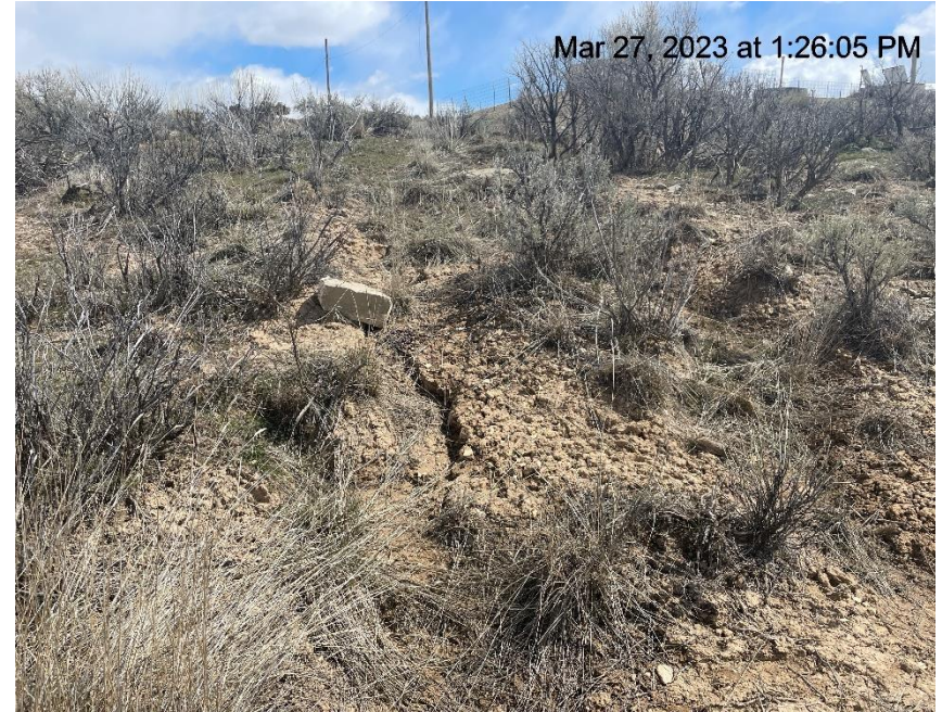
Photo # 3471 Rill erosion on slope
