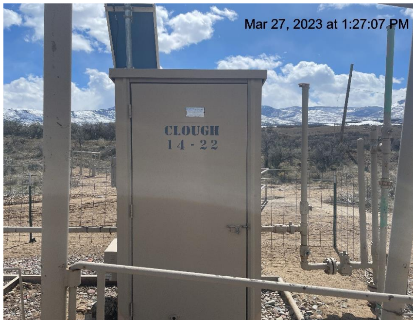
Photo # 3477 Meter calibration info not conspicuously posted
