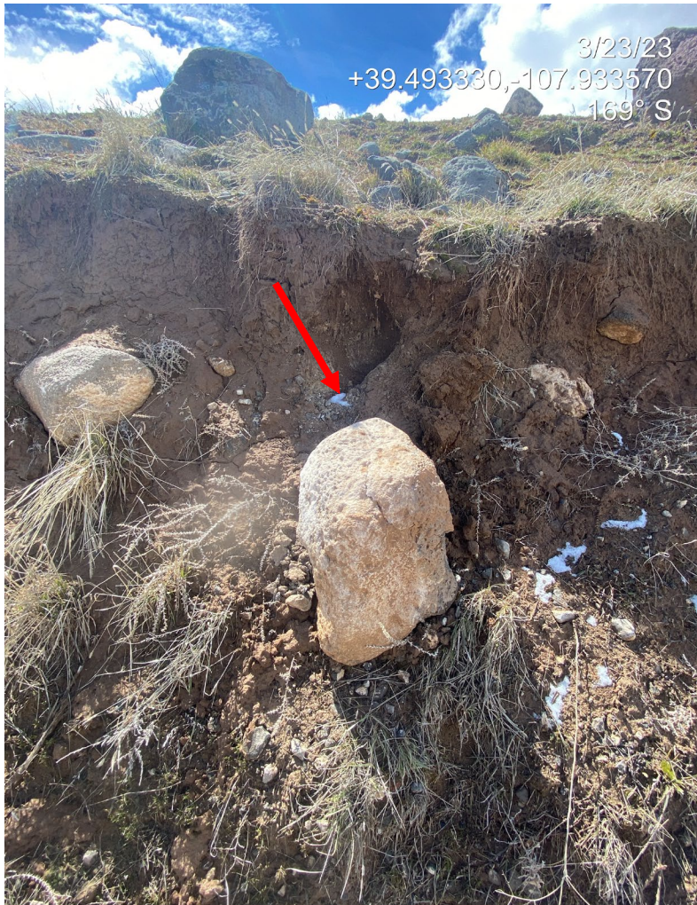
Photo 5. Photos show the unstable, eroding cut slope at the south of the location. Note evidence of recent falling rock, indicating ongoing erosion.
