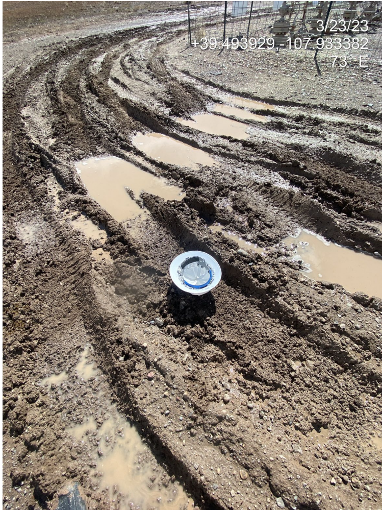
Photo 9. Photo shows lack of pad stabilization.
