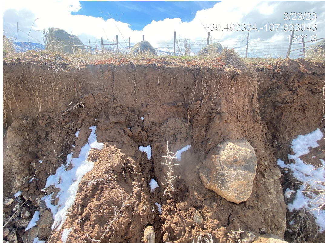
Photo 6. Photos show the cut slope at the south of the location. Note gully and rill erosion and undercutting and exposed roots, indicating the cut is migrating south/back into undisturbed areas.
