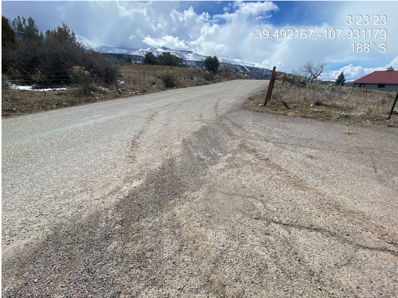
Photo 10. Photo shows tracking onto county road.
