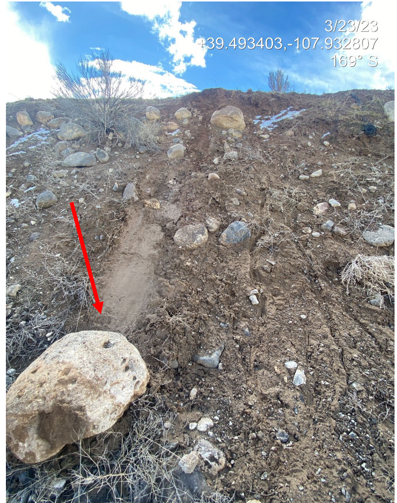
Photo 5. Photos show the unstable, eroding cut slope at the south of the location. Note evidence of recent falling rock, indicating ongoing erosion.
