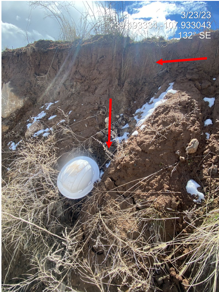
Photo 6. Photos show the cut slope at the south of the location. Note gully and rill erosion and undercutting and exposed roots, indicating the cut is migrating south/back into undisturbed areas.
