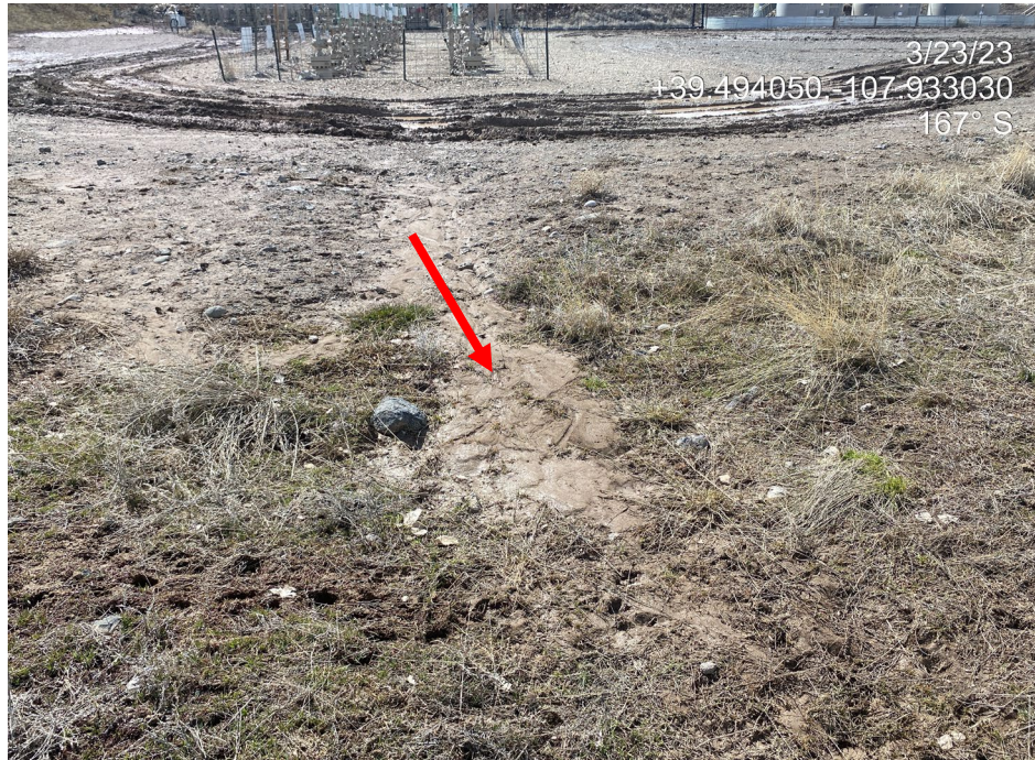
Photo 7. Photo shows sediment runoff from the working pad area into interim areas (left) and from cut slopes/interim areas where rill erosion is occurring onto the pad (right).
