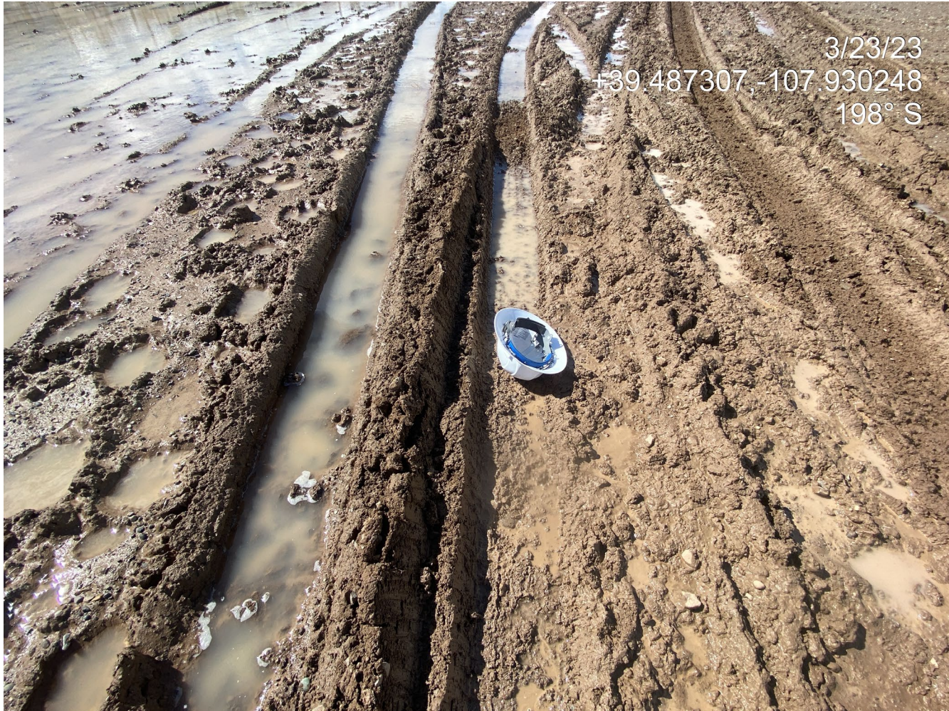
Photo 2. Photo shows lack of pad stabilization.
