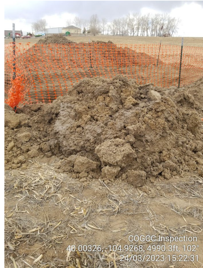
Photo 2 – South Excavation, wet stockpile with hydrocarbon odor and no liner.
