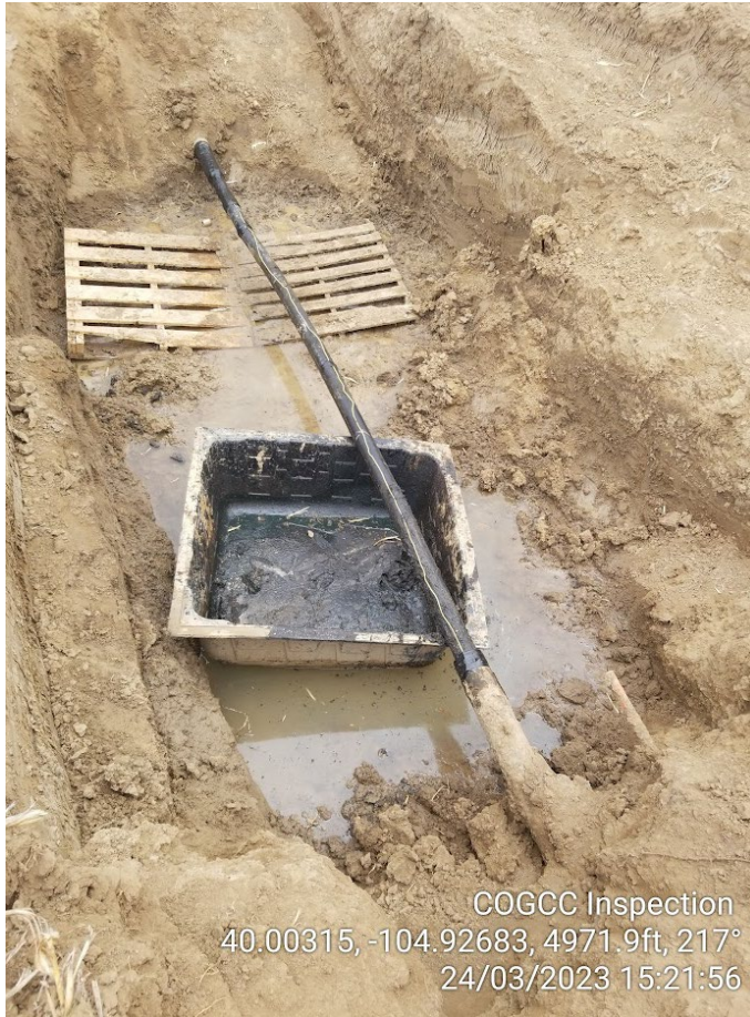
Photo 1 – South Excavation groundwater visible with sheen and flecks of hydrocarbon material.
