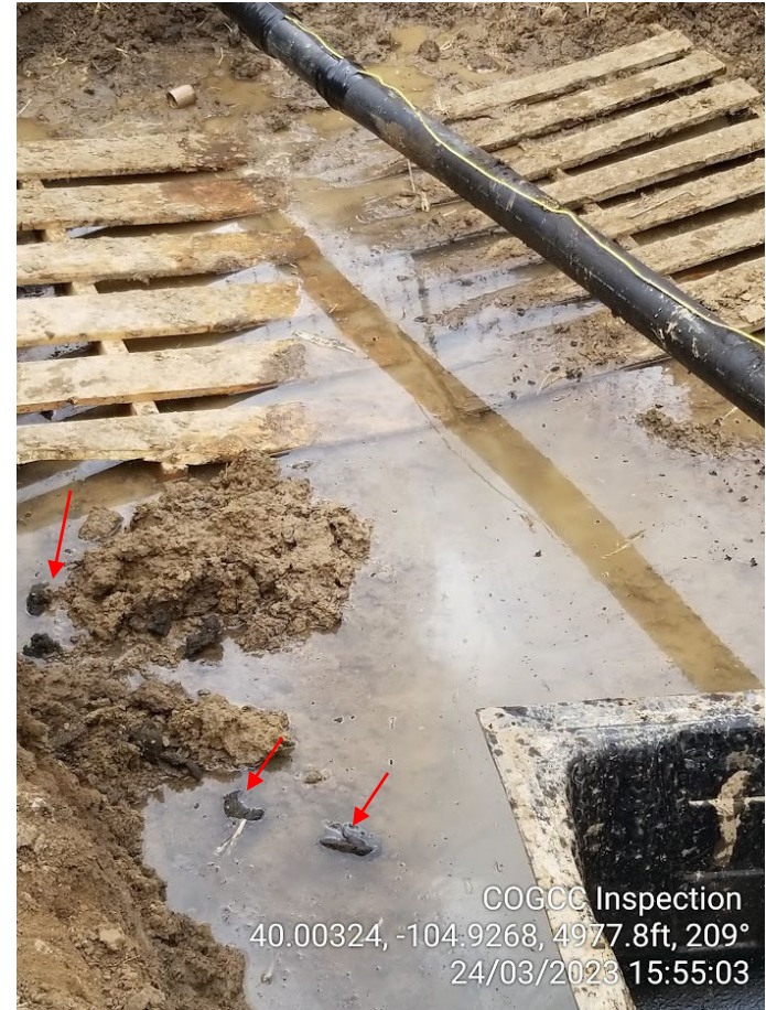
Photo 2 – South Excavation groundwater visible with sheen and flecks of hydrocarbon material. Arrows indicate heavily stained material.
