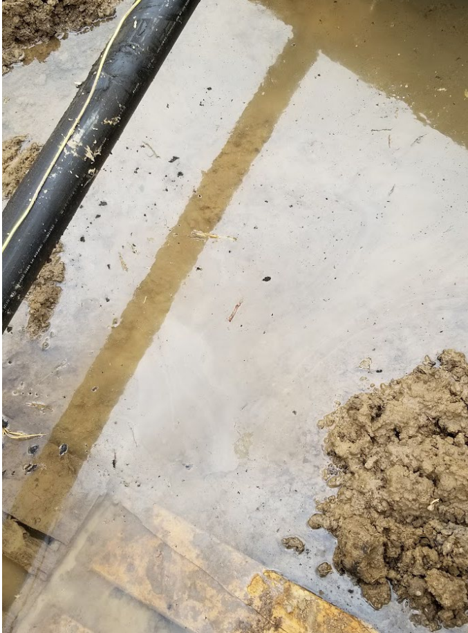
Photo 3 – South Excavation groundwater visible with sheen and flecks of hydrocarbon material.
