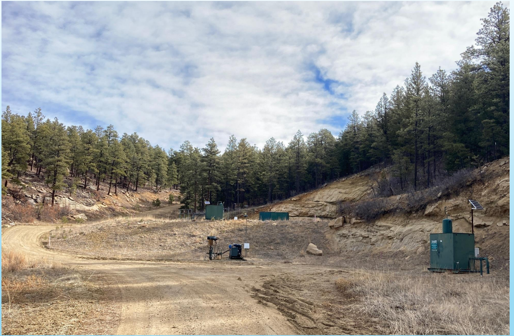
PHOTO 2: ORIGINAL WELL LOCATION
