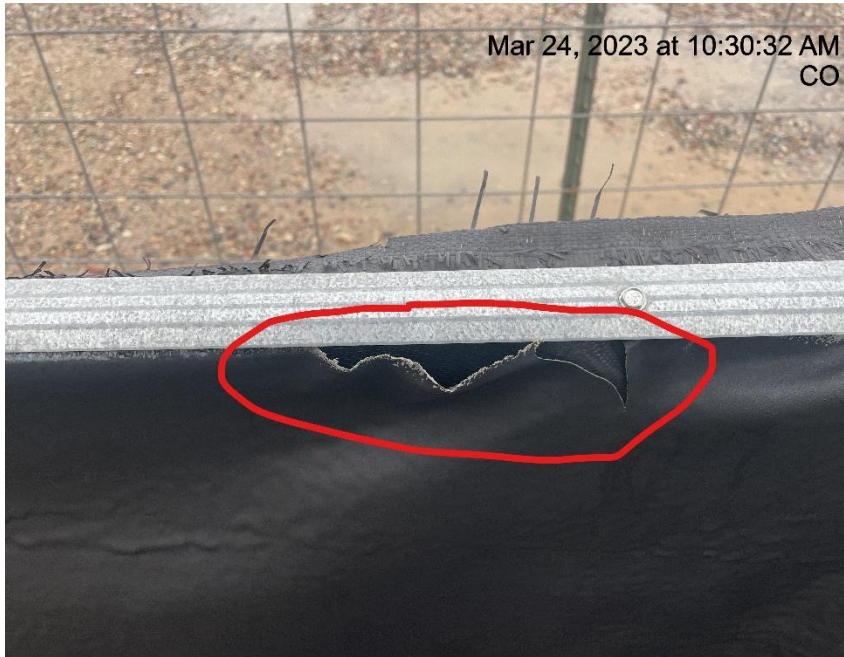
Photo # 3121 Containment needs maintenance
