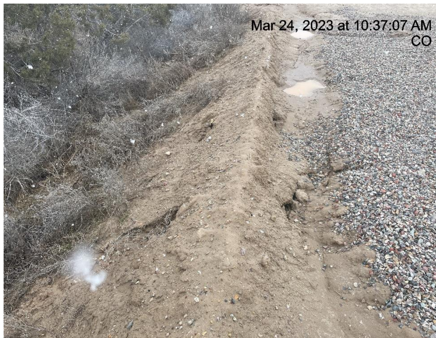
Photo # 3133 Tunnel erosion through berm (east side of pad)
