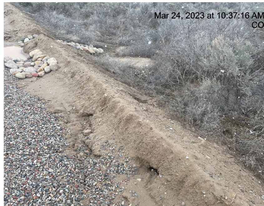
Photo # 3134 Tunnel erosion through berm (east side of pad)
