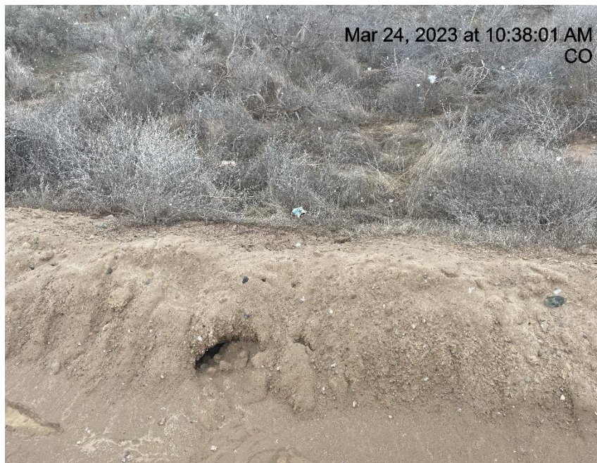
Photo # 3138 Tunnel erosion
