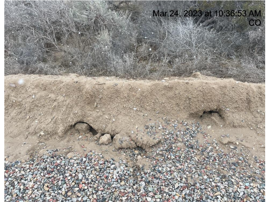
Photo # 3132 Tunnel erosion (east side of pad)
