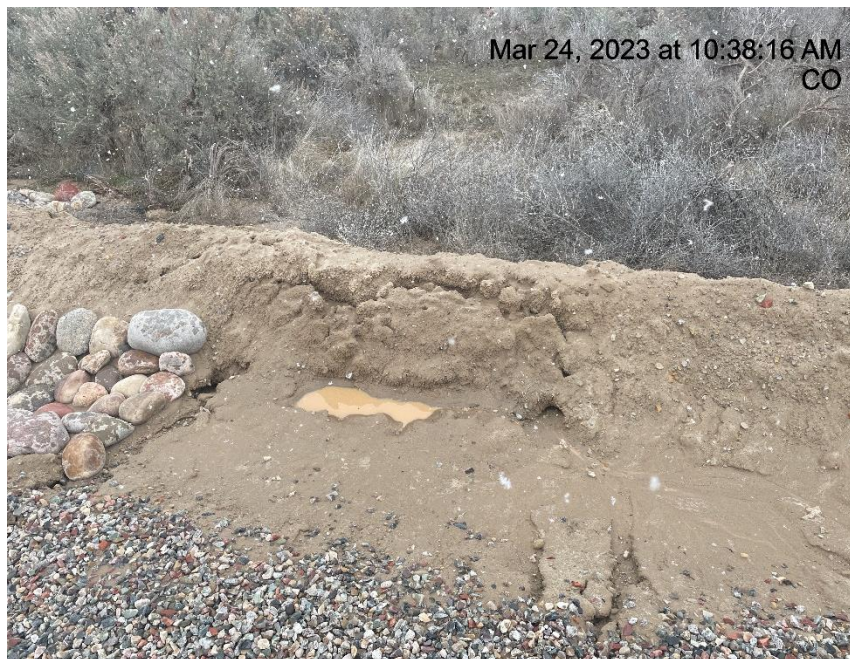
Photo # 3140 Tunnel erosion through berm (east side of pad)
