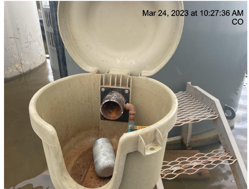
Photo # 3116 Open ended load line
