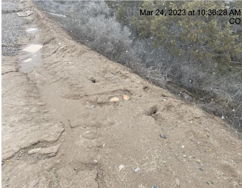
Photo # 3129 Tunnel & Rill erosion on location (east side of pad)
