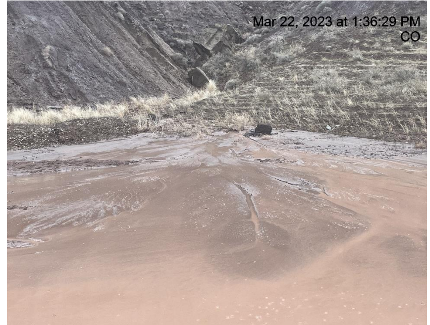
Photo # Insufficient run on controls/BMP's
