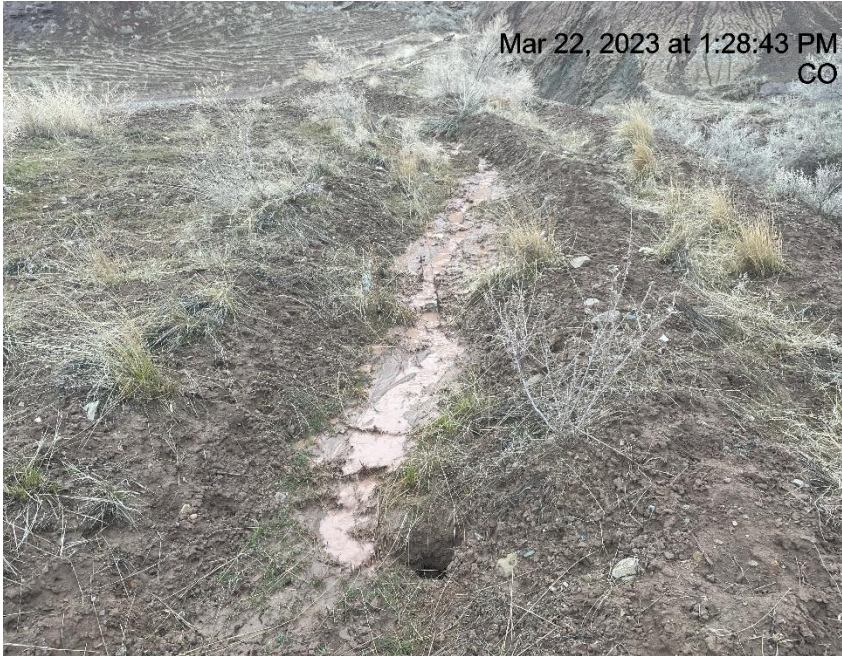
Photo # 2845 Tunnel erosion/ditch needs maintenance (upper tier of pad, east side)
