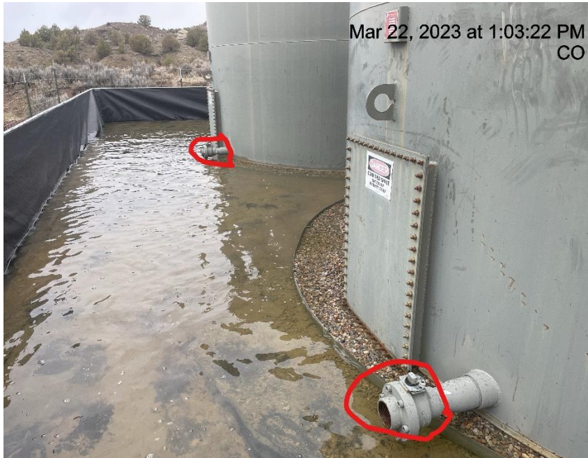
Photo # 2821 Open ended load lines
