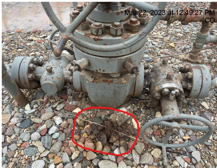
Photo # 2808 Stained soils & gravel in front of SG 342-28 wellhead
