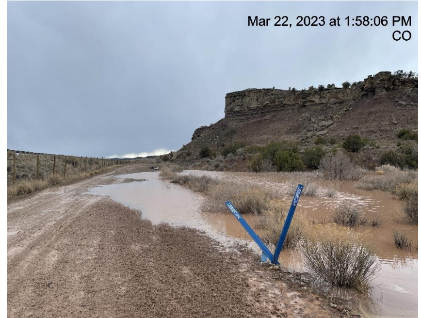
Photo # 2890 Insufficient run on controls/BMP's/ & degradation of roadway (4/10 th of a mile down lease road)
