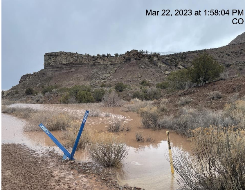
Photo # 2889 Insufficient run on controls/BMP's/ & degradation of roadway (4/10 th of a mile down lease road)
