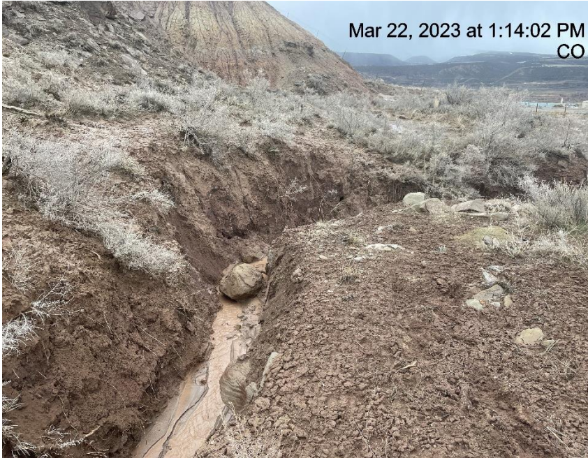
Photo # 2831 Erosion/ditch needs maintenance (lower tier of pad east side)
