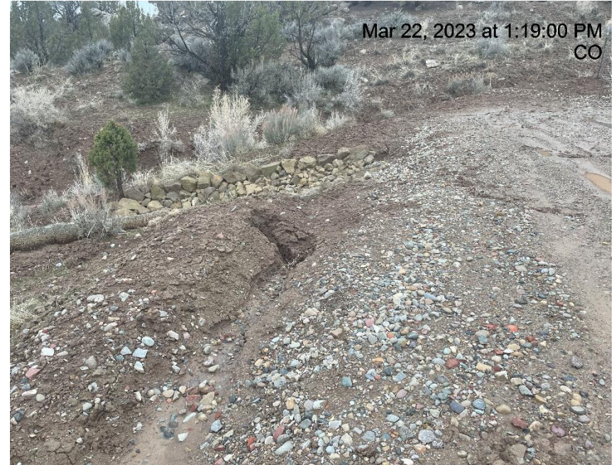
Photo # 2836 Erosion/ditch needs maintenance (upper tier of pad, SW corner near rip rap run)
