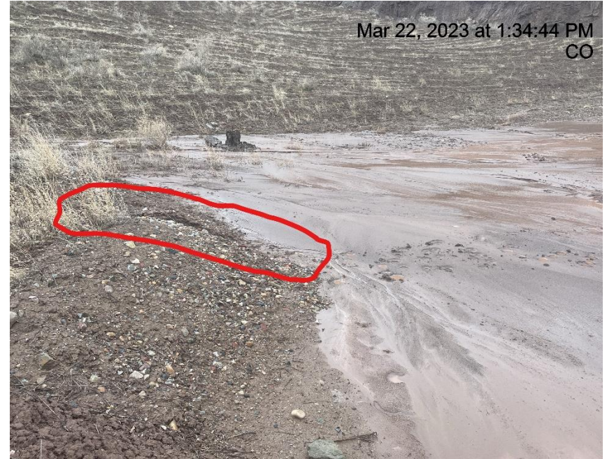
Photo # 2865 Berm needs maintenance (upper tier of past NW side)
