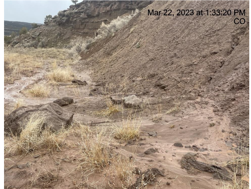
Photo # 2860 Insufficient run on controls/BMP's/sediment encroaching on habitat & choking of vegetation
