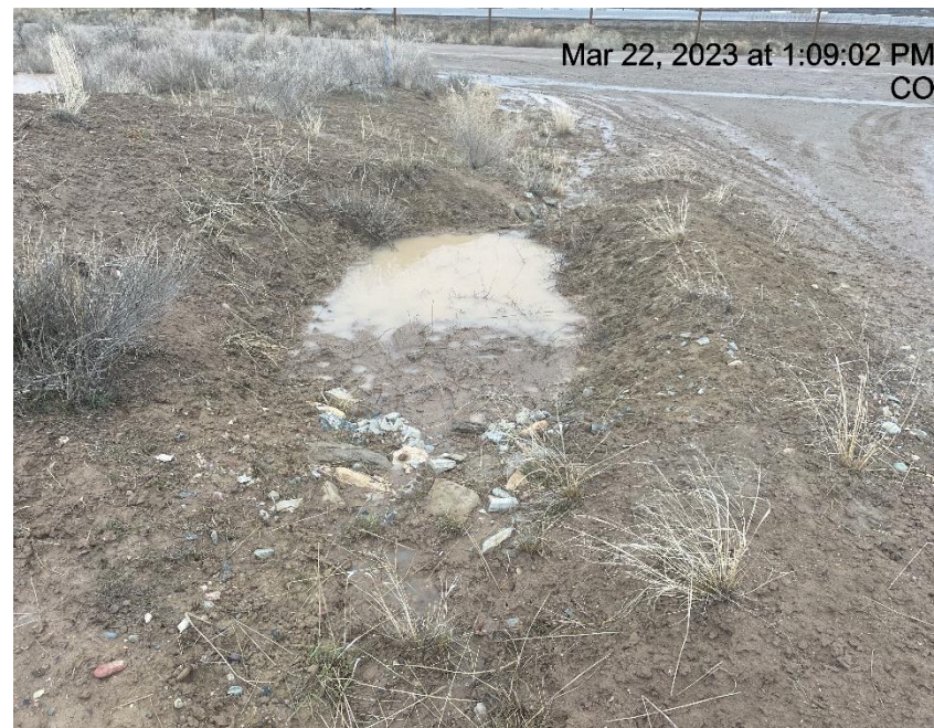
Photo # 2822 Sediment trap needs maintenance (near entrance to spur road)
