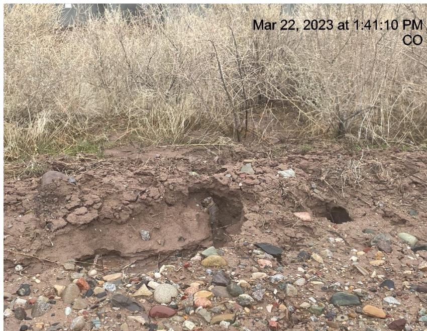
Photo # 2887 Rill & tunnel erosion (upper tier of pad, south side)
