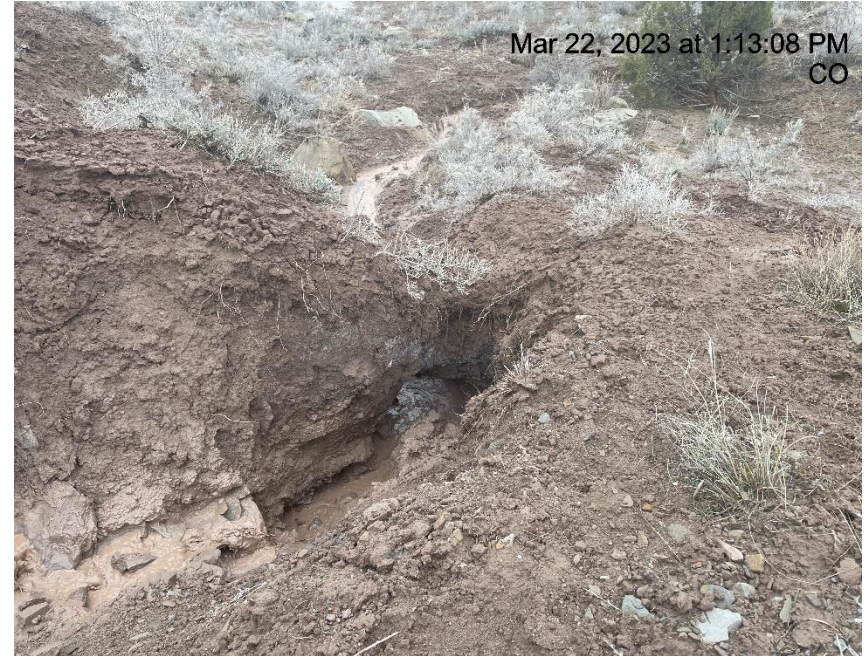
Photo # 2828 Erosion/ditch needs maintenance (lower tier of pad east side)
