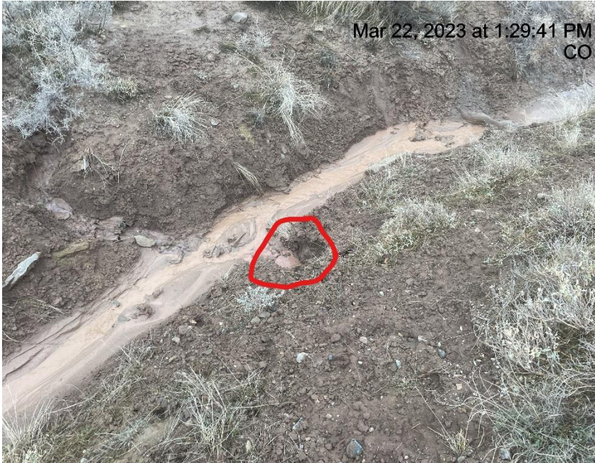
Photo # 2850 Tunnel erosion/berm needs maintenance (upper tier of pad, east side)
