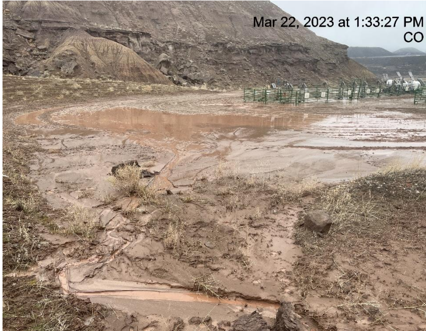
Photo # 2861 Insufficient run on controls/BMP's
