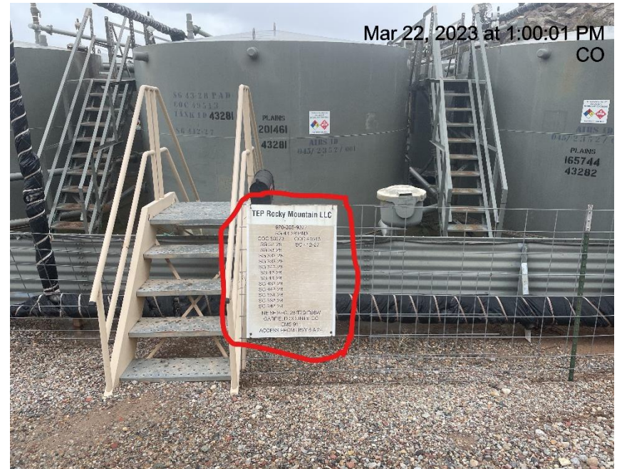
Photo # 2816 Battery sign missing required information
