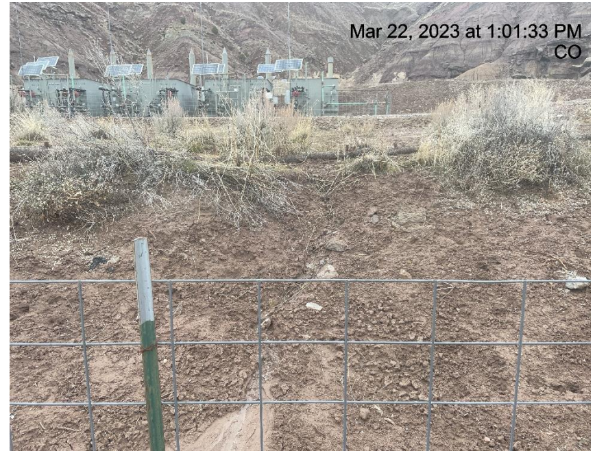
Photo # 2818 Waddles need maintenance/rill erosion/sediment encroaching on equipment
