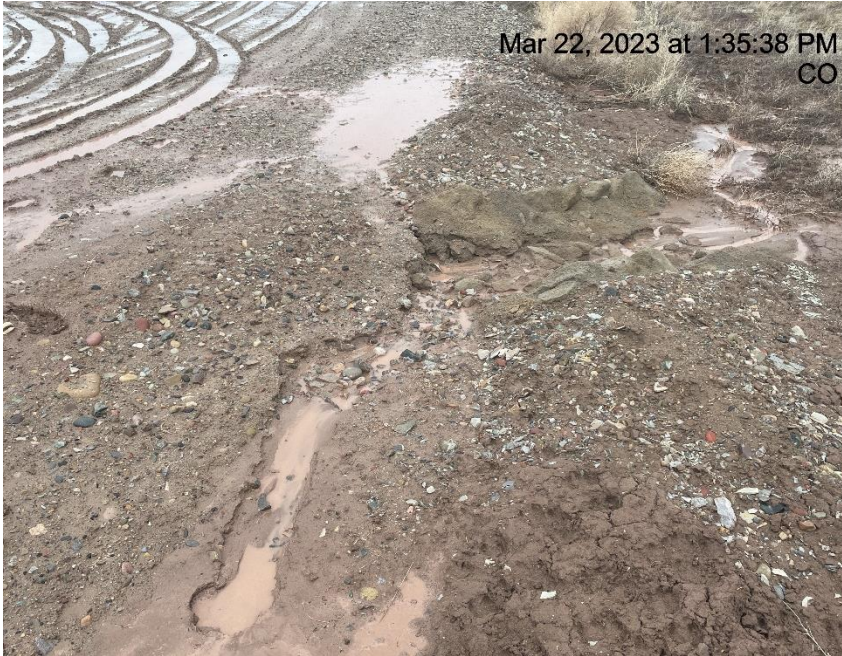
Photo # 2871 Rill erosion/rip rap needs maintenance (upper tier, west side)
