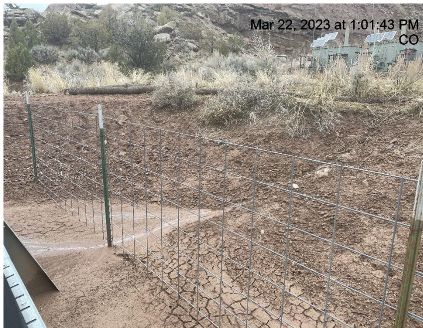
Photo # 2819 Waddles need maintenance/rill erosion/sediment encroaching on equipment
